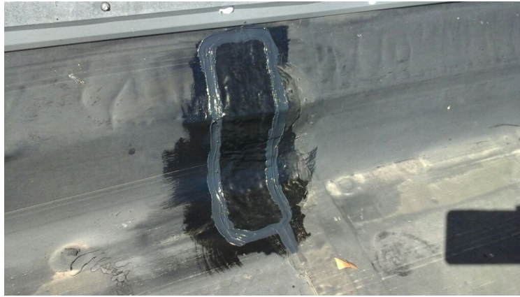
Photo showing a repair made to the perimeter flashing.
