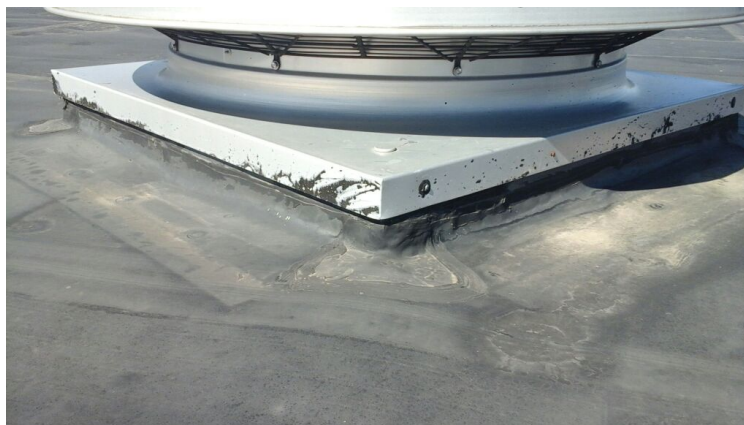
Photo showing condition of projection flashings.
