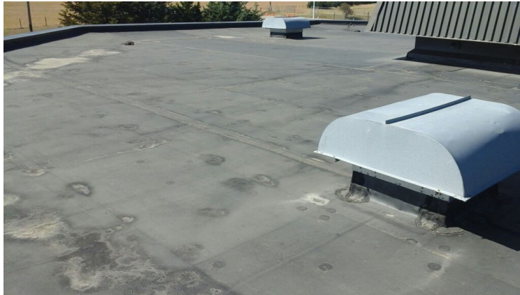
Photo showing overview of Area 03 Roof.
