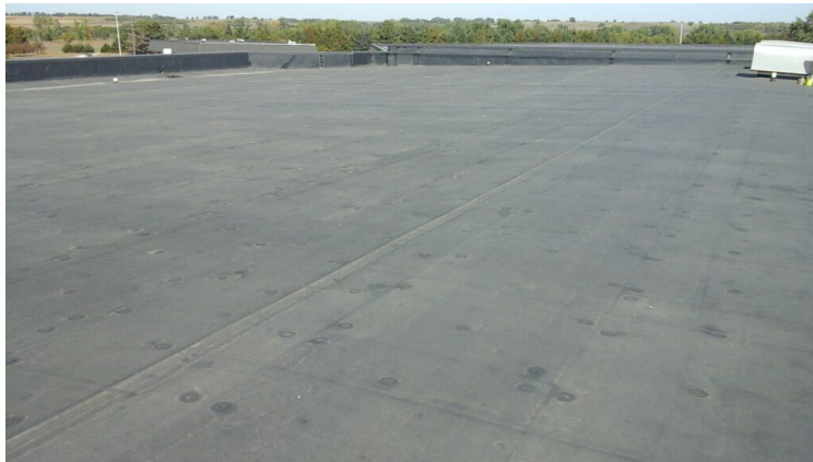
Photo showing additional overview of Area 05 Roof.
