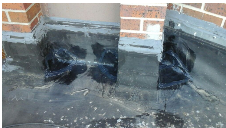
Photo showing repairs made to the perimeter flashings.
