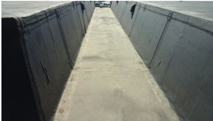
Photo showing additional overview of Area 10 Roof.
