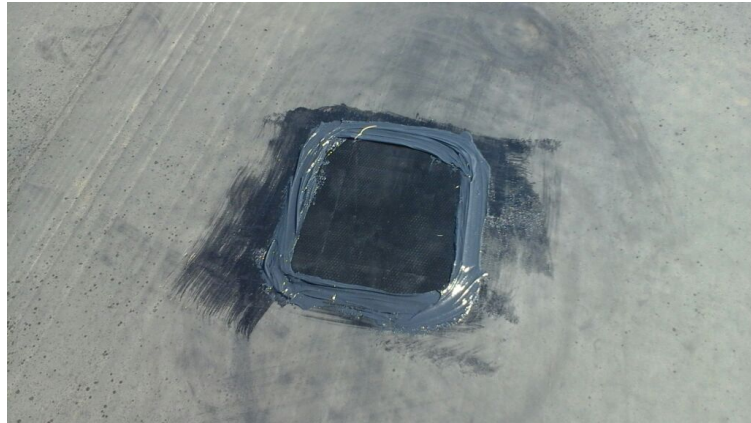
Photo showing repair made to the field membrane.
