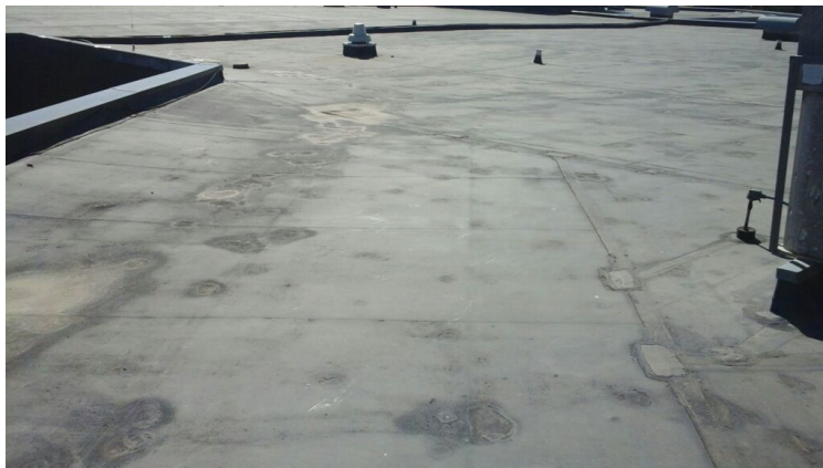
Photo showing additional overview of Area 04 Roof.
