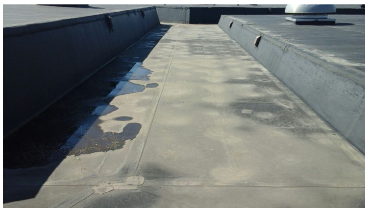
Photo showing additional overview of Area 10 Roof.
