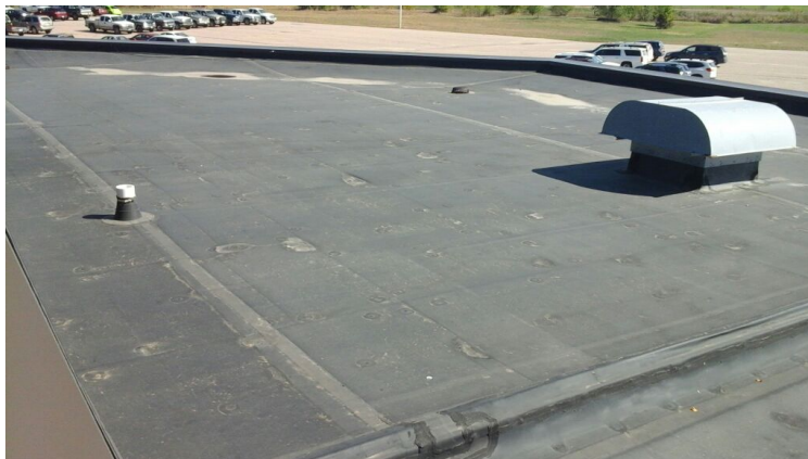
Photo showing additional overview of Area 01 Roof.
