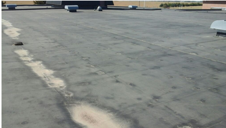
Photo showing overview of Area 02 Roof.
