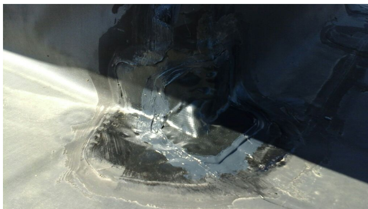
Photo showing repair made to the projection flashing.
