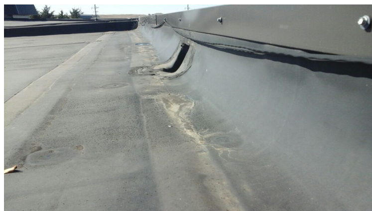
Photo showing condition of the perimeter flashings.
