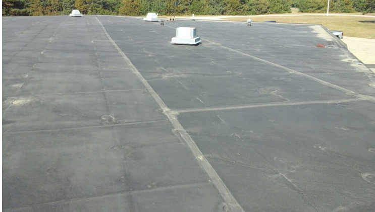
Photo showing overview of Area 11 Roof.
