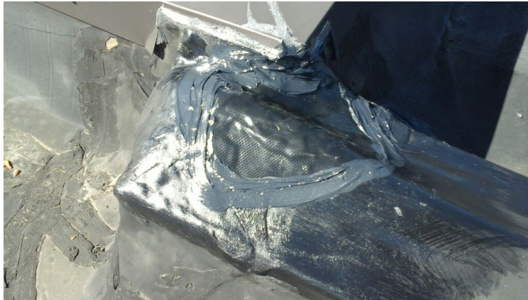
Photo showing repair made to the expansion joint.
