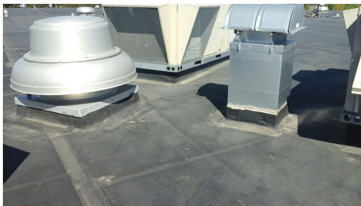
Photo showing condition of projection flashings.
