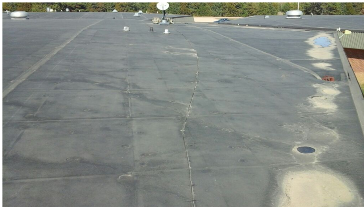
Photo showing additional overview of Area 08 Roof.
