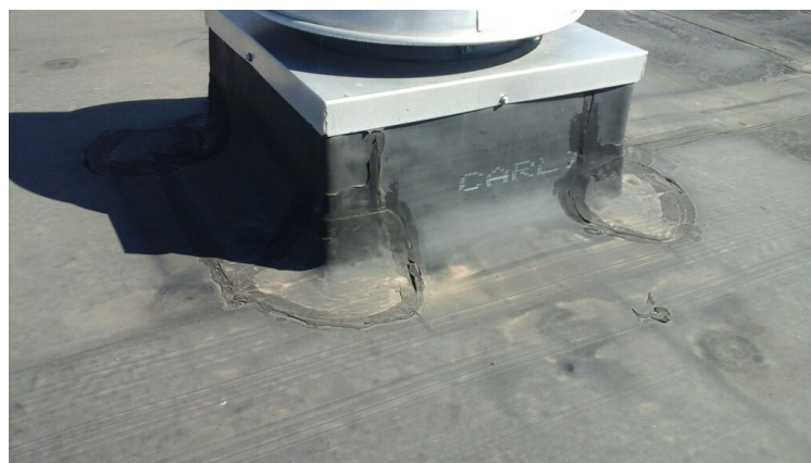
Photo showing condition of projection flashings.
