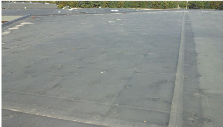
Photo showing overview of Area 06 Roof.
