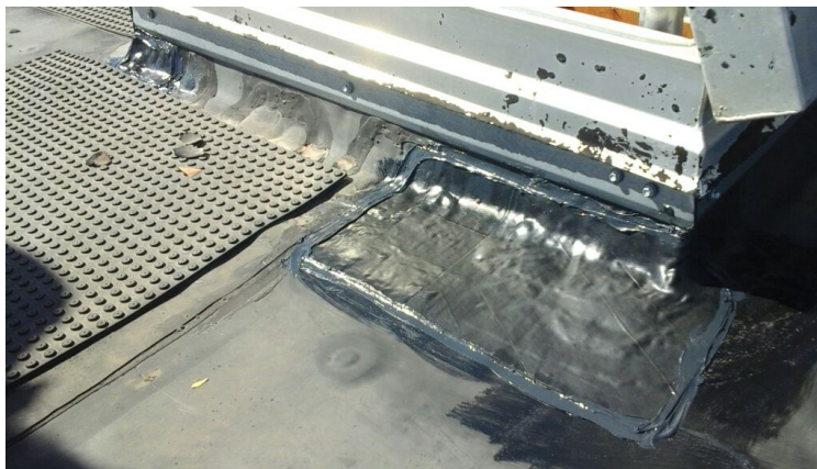
Photo showing repairs made to hatch flashings.
