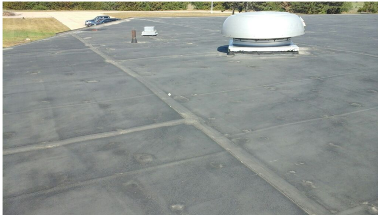
Photo showing additional overview of Area 09 Roof.
