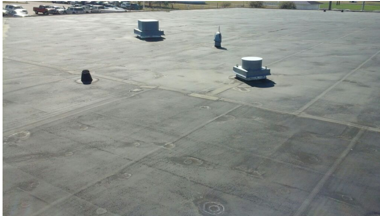
Photo showing overview of Area 12 Roof.
