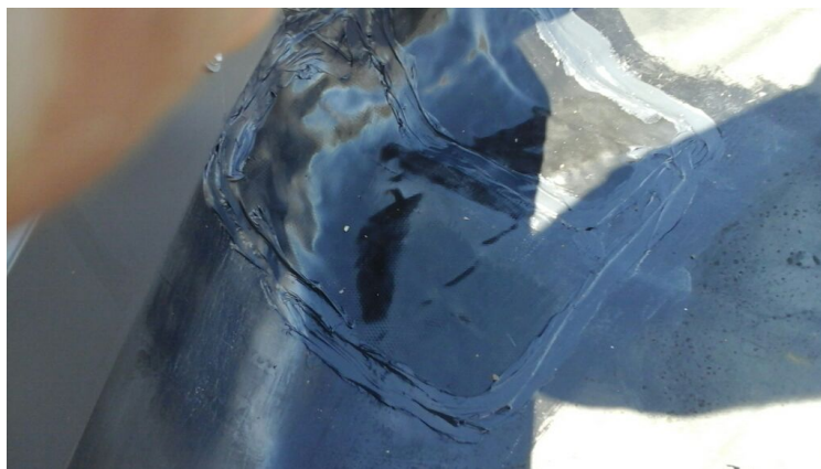
Photo showing repair made to the perimeter flashing.
