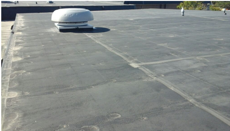
Photo showing additional overview of Area 11 Roof.
