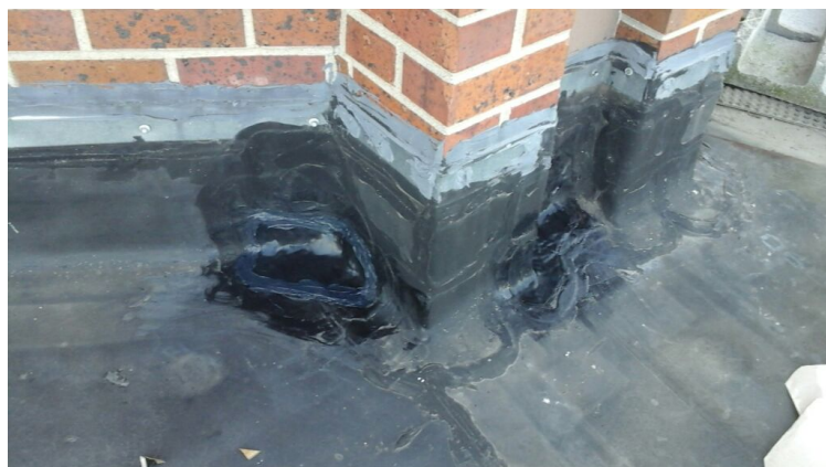
Photo showing repairs made to the perimeter flashing.
