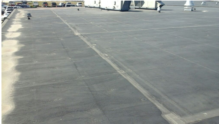
Photo showing overview of Area 08 Roof.
