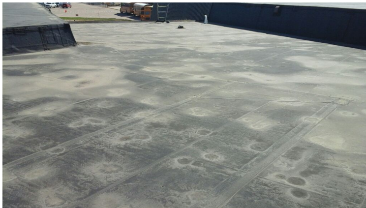
Photo showing additional overview of Area 10 Roof.
