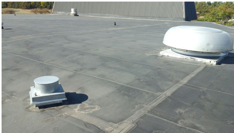
Photo showing additional overview of Area 12 Roof.
