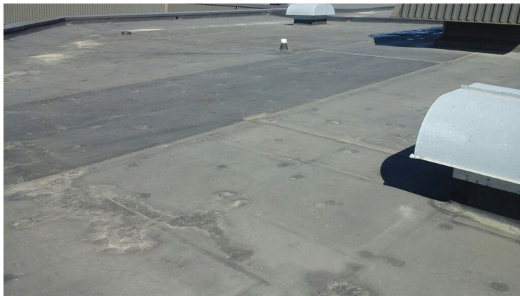
Photo showing additional overview of Area 03 Roof.
