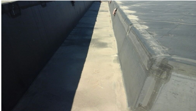
Photo showing additional overview of Area 10 Roof.
