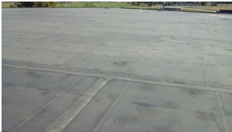
Photo showing additional overview of Area 06 Roof.
