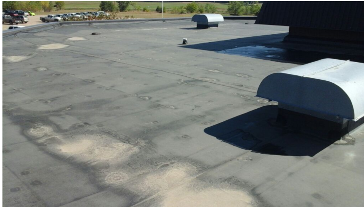
Photo showing overview of Area 01 Roof.
