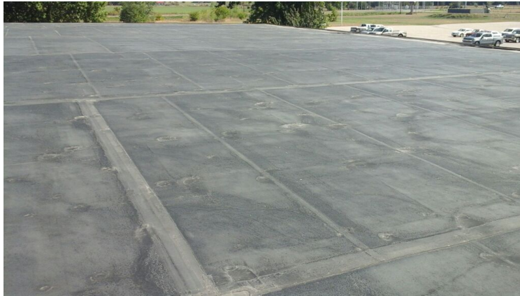
Photo showing overview of Area 09 Roof.
