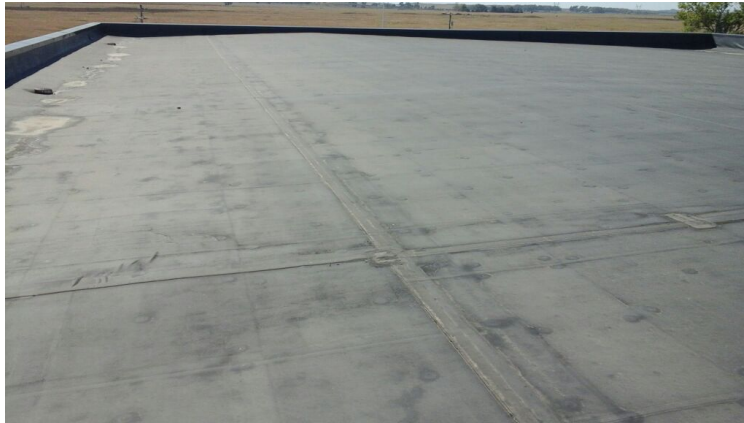
Photo showing overview of Area 05 Roof.
