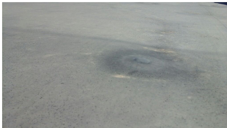
Photo showing fasteners backing out under field membrane.
