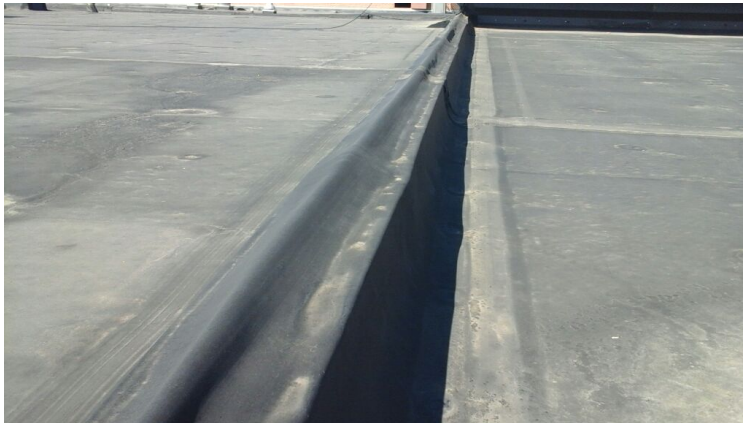
Photo showing condition of the expansion joint.
