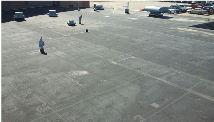
Photo showing overview of Area 07 Roof.
