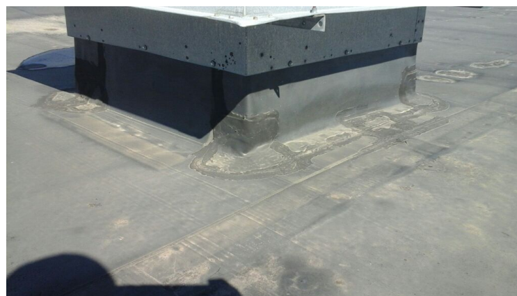
Photo showing condition of projection flashings.
