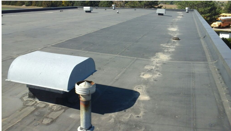
Photo showing overview of Area 13 Roof.
