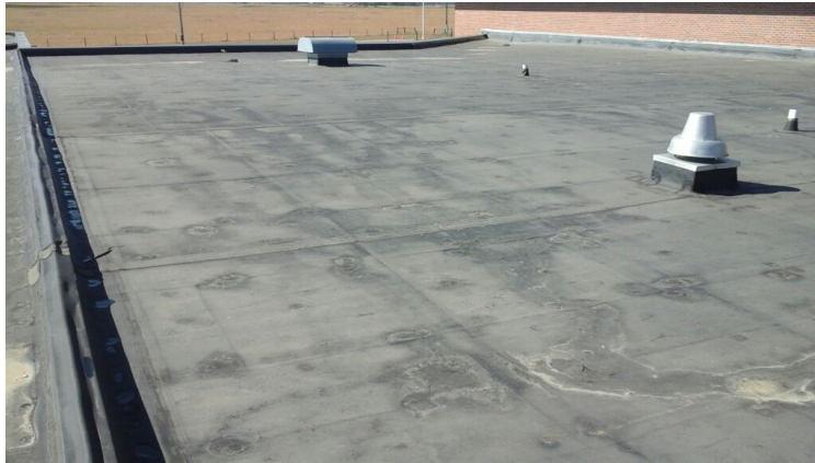
Photo showing overview of Area 04 Roof.
