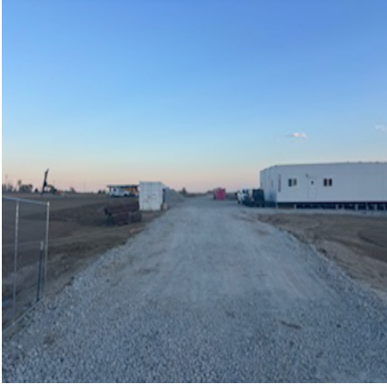
Figure 1 South Entrance to Work Trailer
