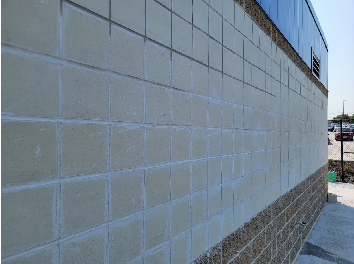
Bennington HS Stadium Improvements
