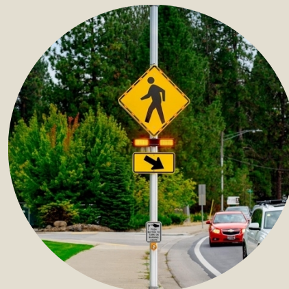
Rectangular Rapid Flashing Beacons (RRFBs)
