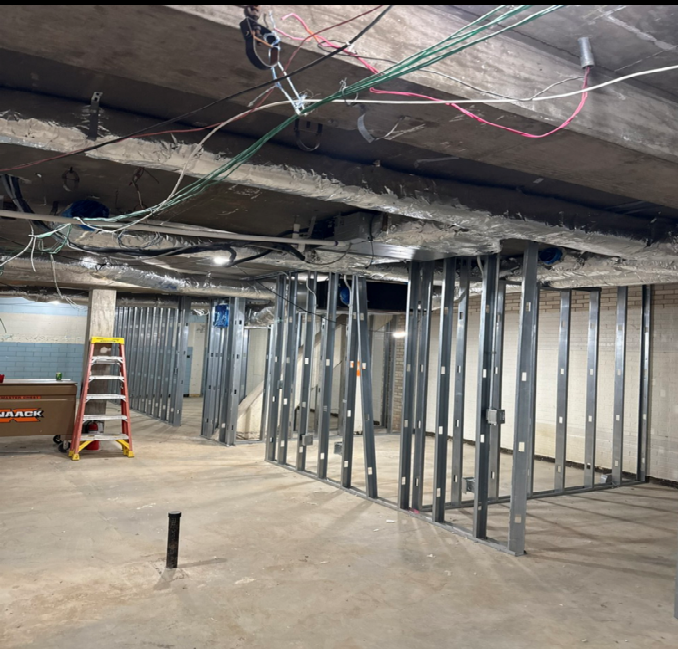
RBE FRAMING - INTERIOR
