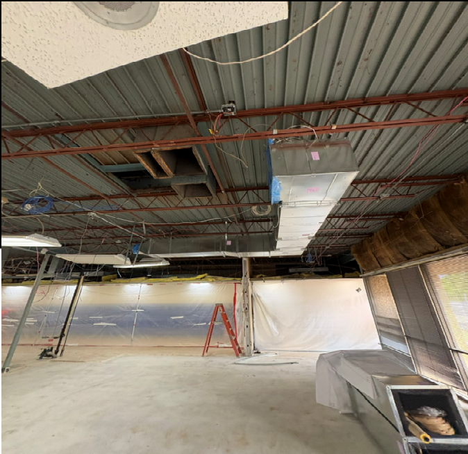
ADMIN CEILING ROUGH-IN
