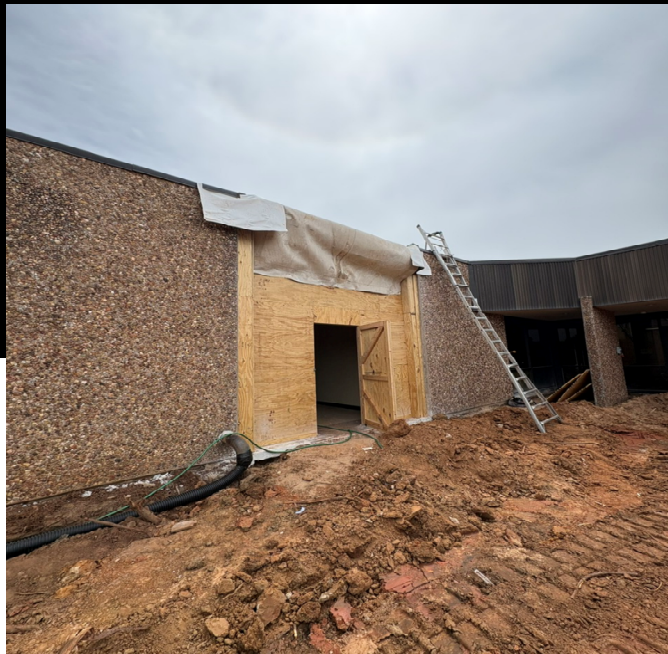
CAFETERIA TEMP PROTECTION
