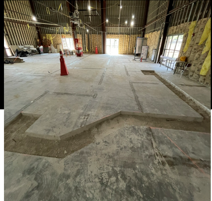
SLAB TRENCH AND WALL LAYOUT
