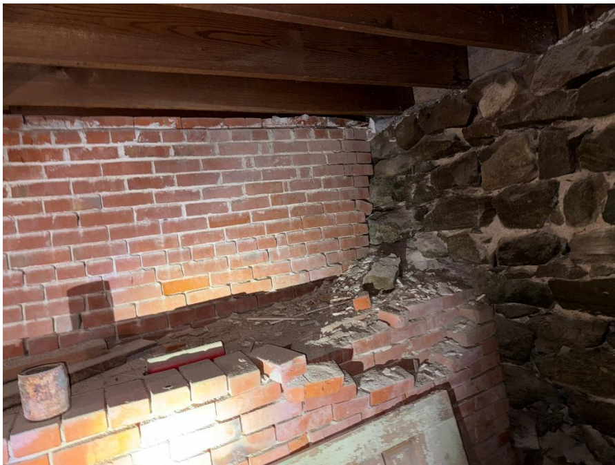
Photo 10 - Basement looking southeast.
