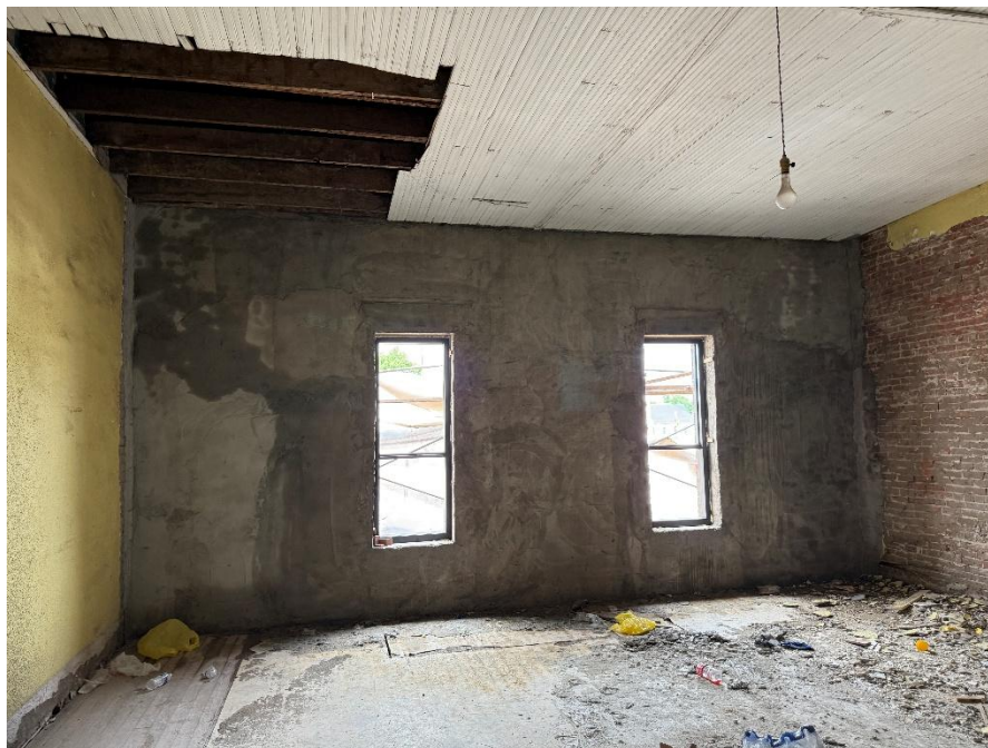
Photo 4 - Coated west second floor wall.
