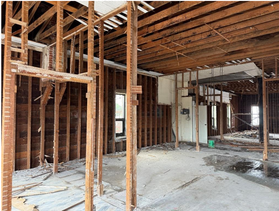
Photo 7 - Second floor wall framing.
