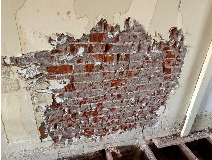
Photo 1 - Plaster removal at north face of intermediate first floor brick wall.
