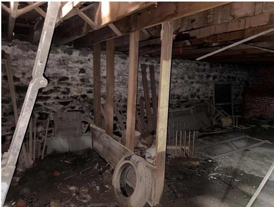
Photo 12 - North basement wall.
