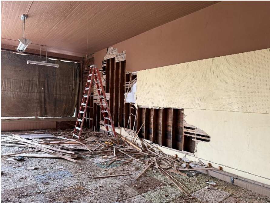
Photo 5 - East end of south first floor wall.
