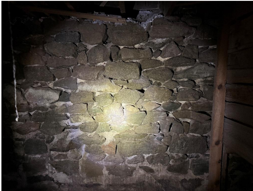
Photo 13 - South basement wall.
