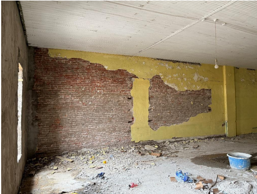
Photo 3 - Plaster removal at second floor north wall.
