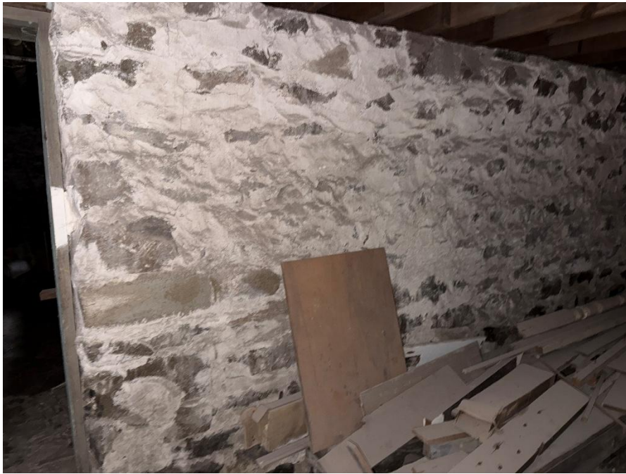
Photo 11 - Interior stone wall.
