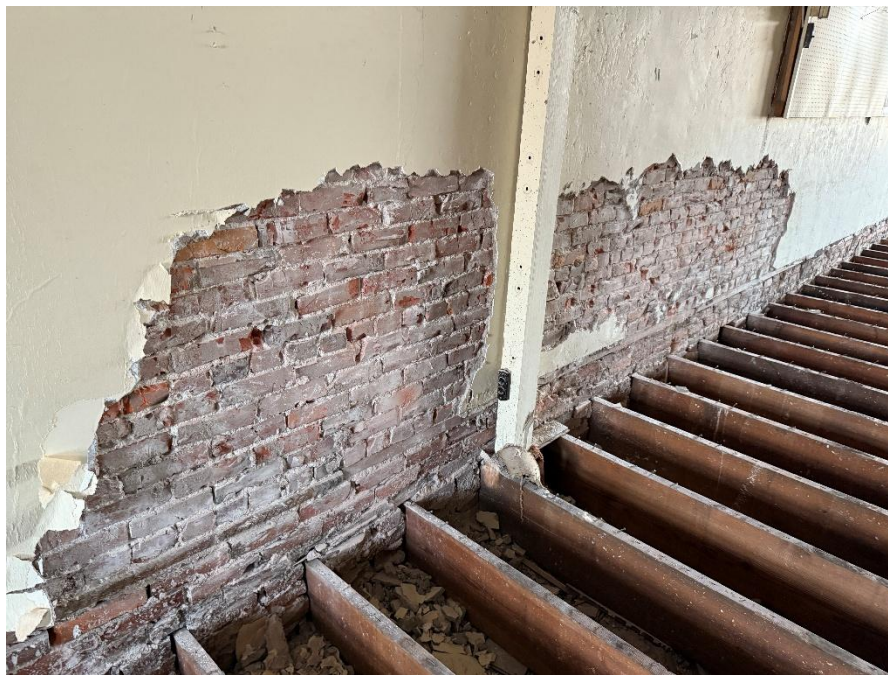
Photo 2 - Plaster removal at first floor north brick wall.
