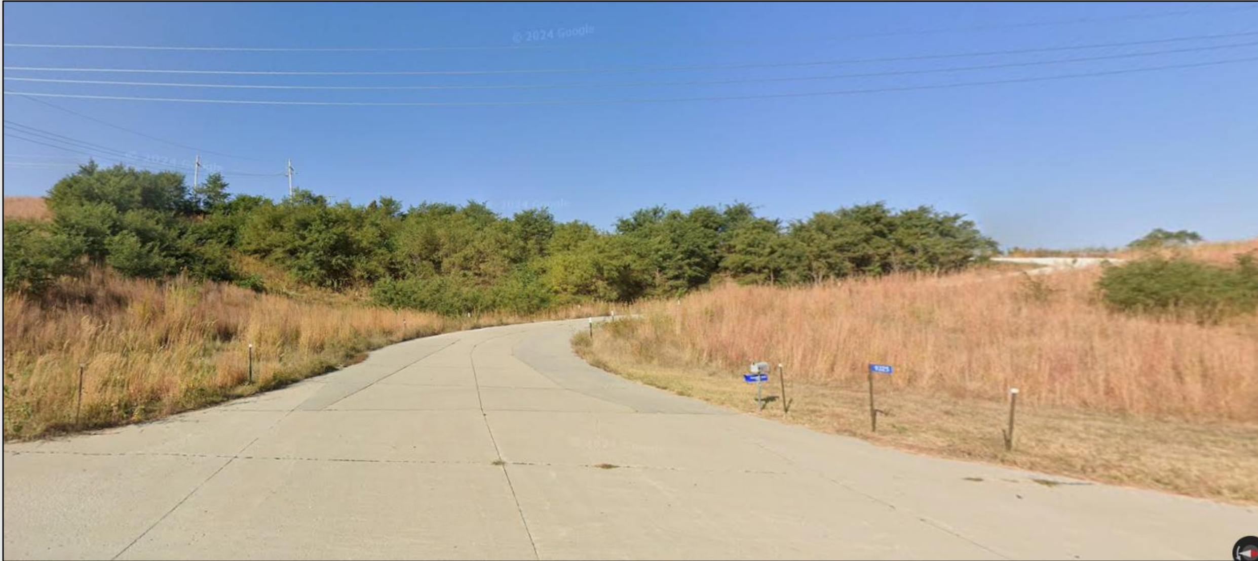
9325 STATE HWY 133 - Preconstruction Soderberg
