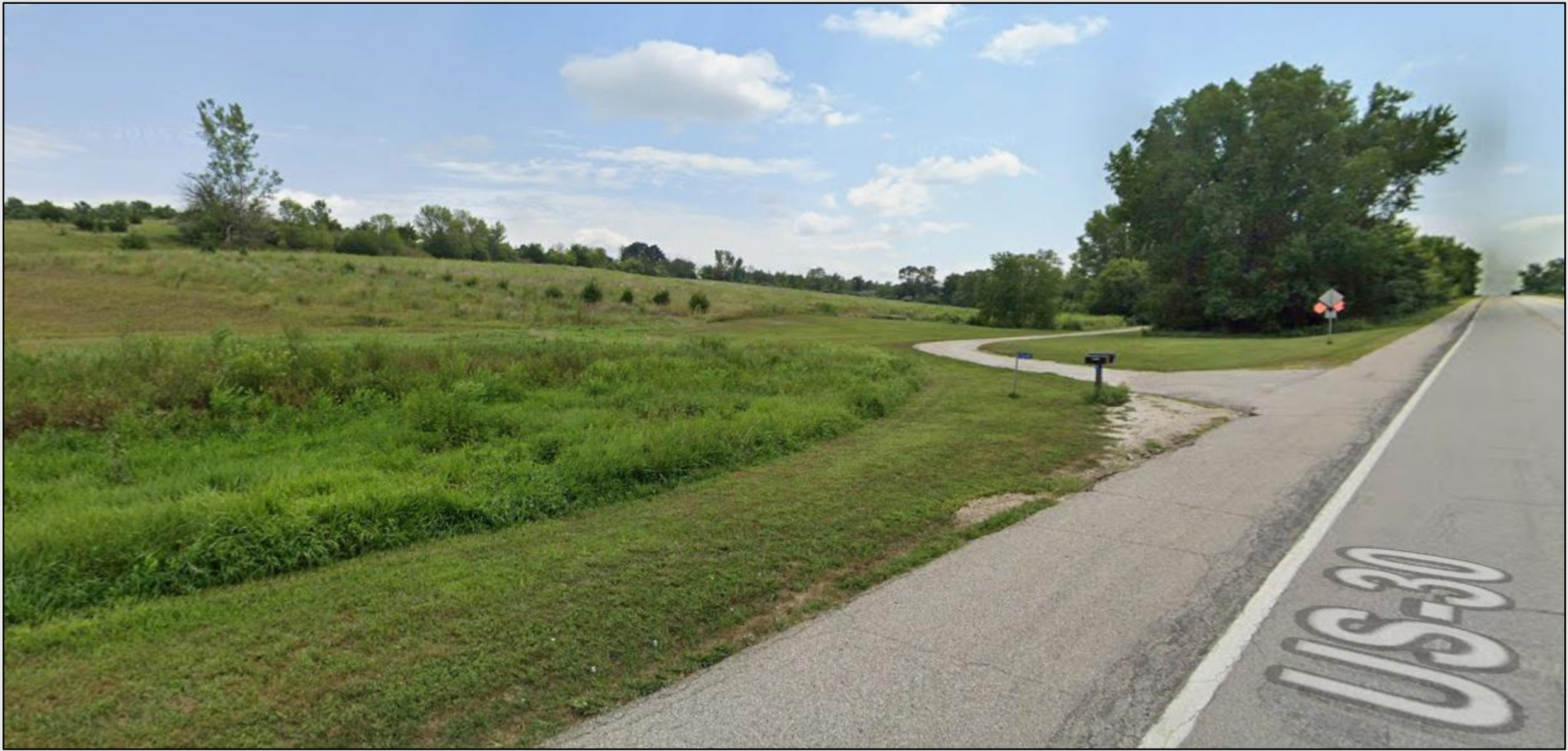
12645 S HWY 30 - Preconstruction Soderberg
