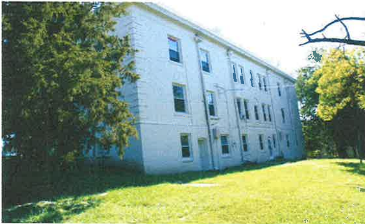
Third building, most North, back (west) to Madison St, circa. 2013,
