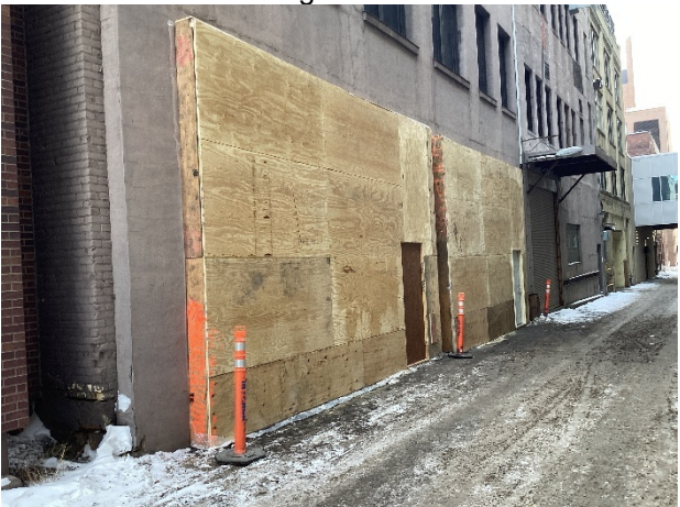
Exterior Wall Temporary Enclosure
