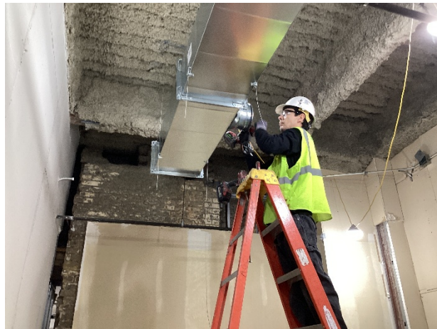
Mechanical Duct Installation
