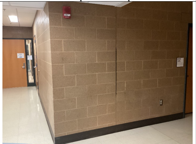
Missing sealant
