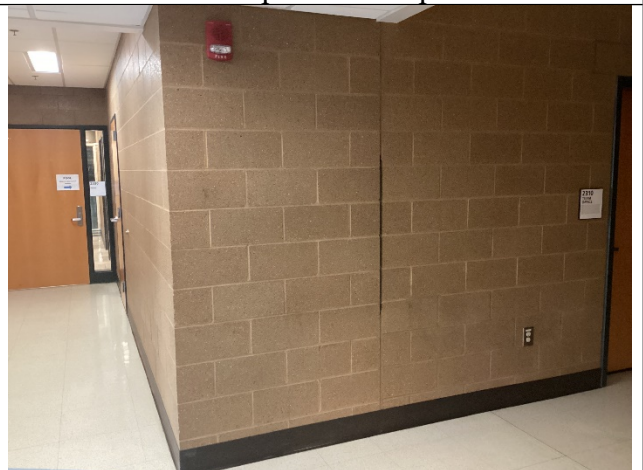
Missing sealant
