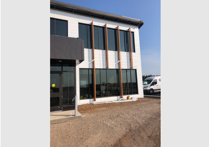
Description Exterior Paneling - DSC Lobby Area
