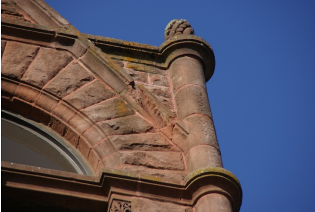
Photo 9: Deteriorated stone
