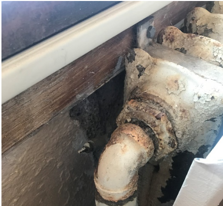
Photo 3 Active Pneumatic Controls
