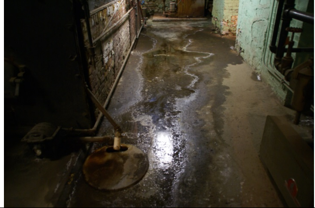
Photo 2: Boiler room floor
