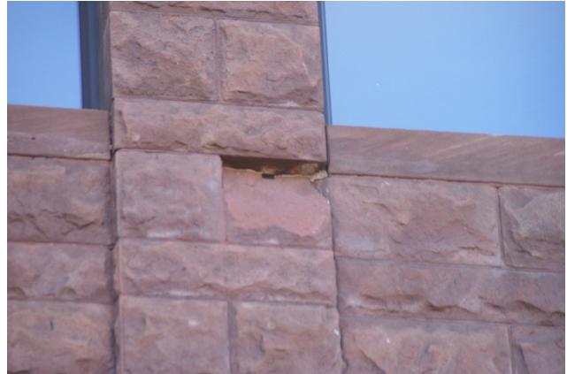
Photo 12: Spalled stone
