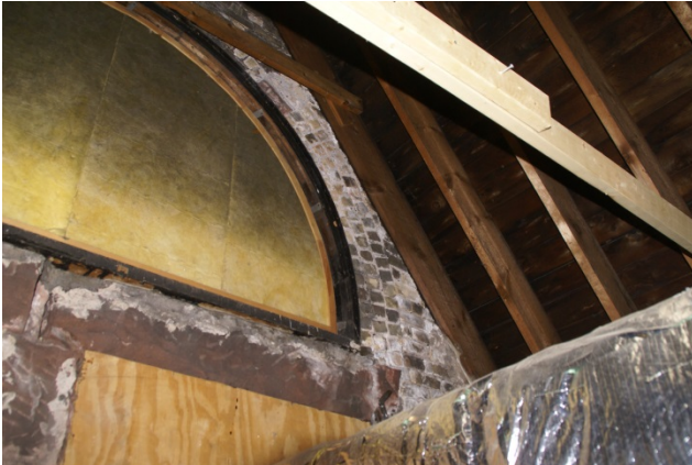
Photo 5: West Turret attic space
