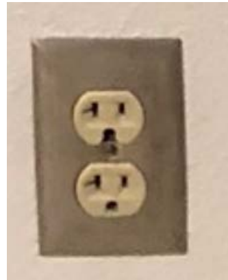
Photo 4: Broken Receptacle
