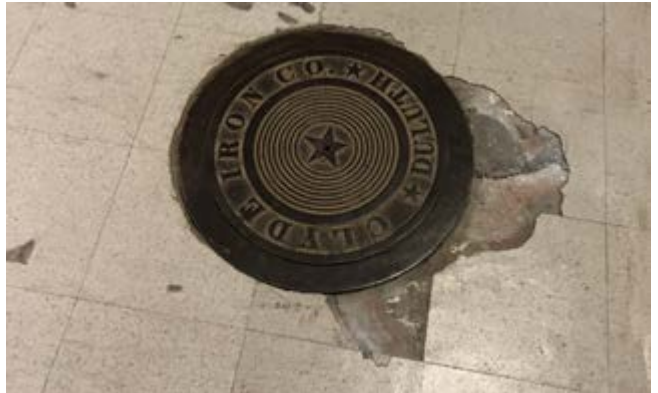
Photo 4 VCT ( Vinyl Composition Tile) Basement
