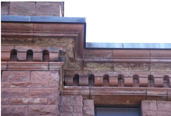
Photo 17: Efflorescence
