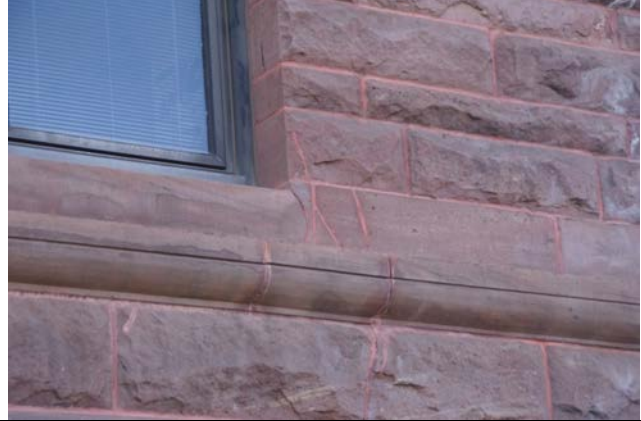
Photo 8: Cracked stone
