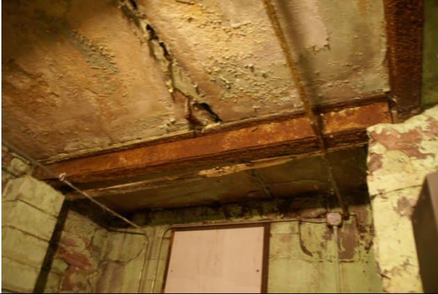
Photo 1: Below main entrance plaza
