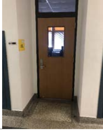
Photo 8 Interior door entrance clearances
