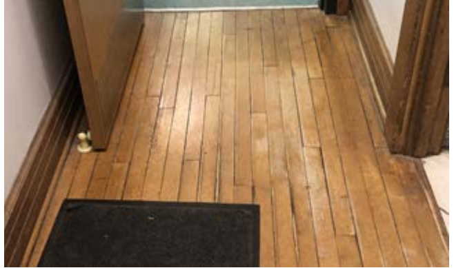
Photo 2 Original wood floor
