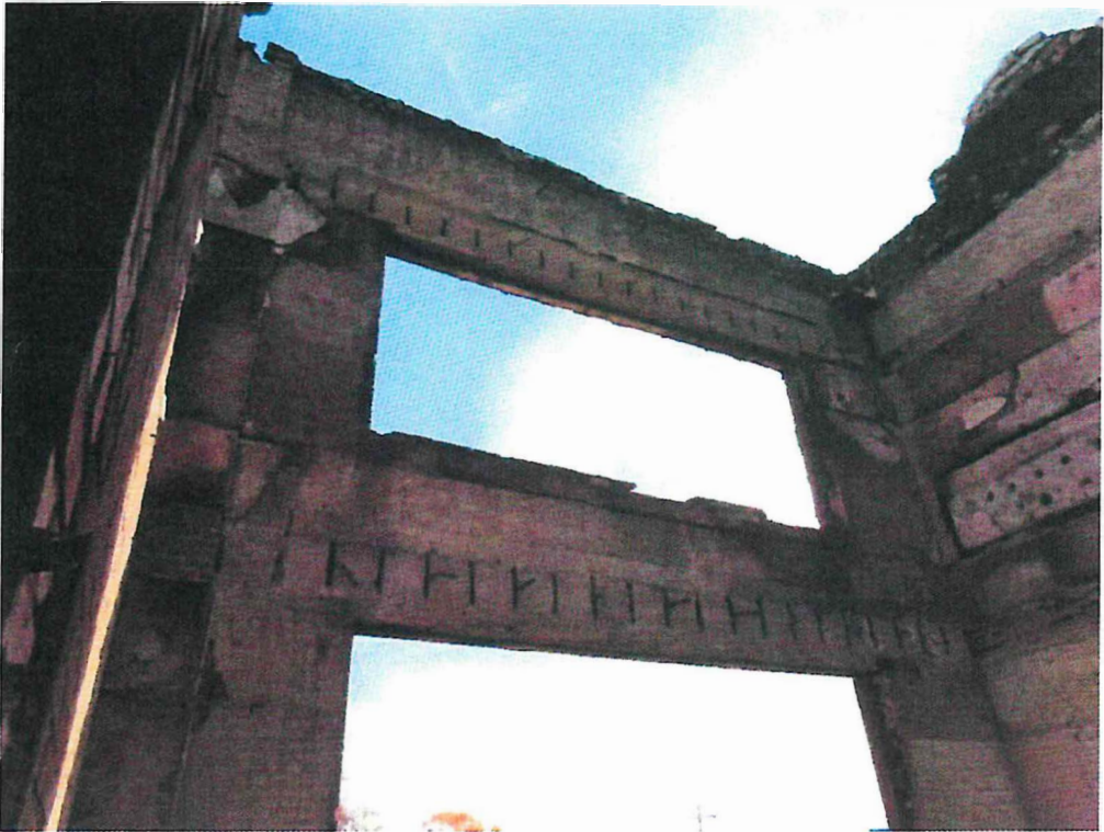
Photograph 6 – MWISD Fanning Building – Concrete Beams Above Windows
