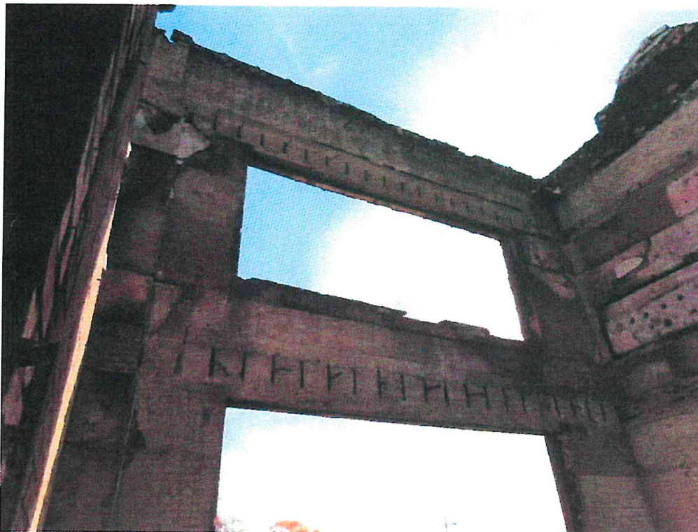
Photograph 6 – MWISD Fanning Building – Concrete Beams Above Windows
