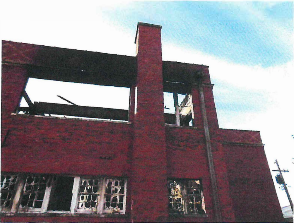
Photograph 5 – MWISD Fanning Building – North Wall
