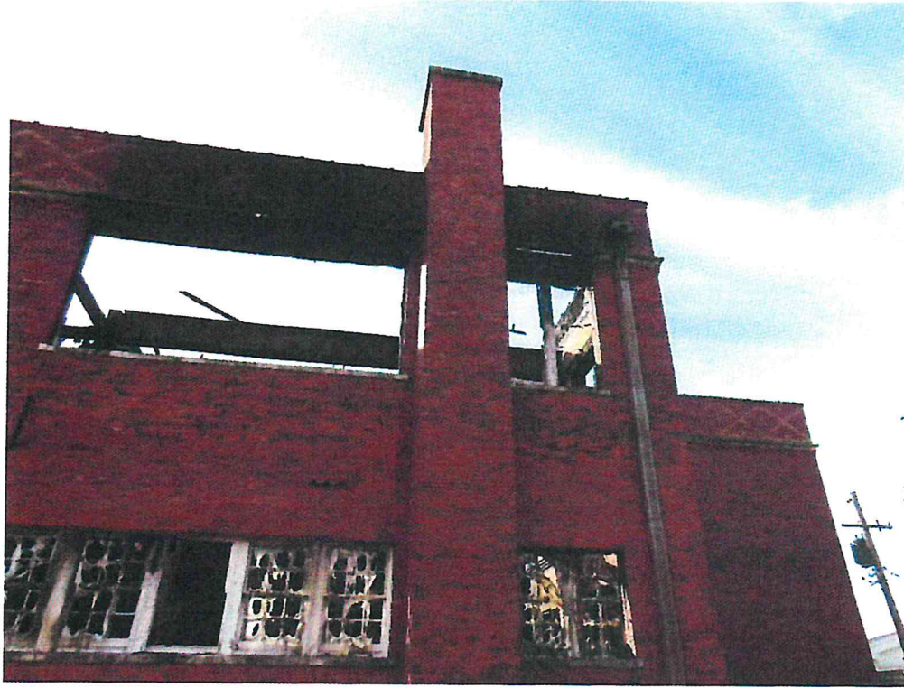
Photograph 5 – MWISD Fanning Building – North Wall
