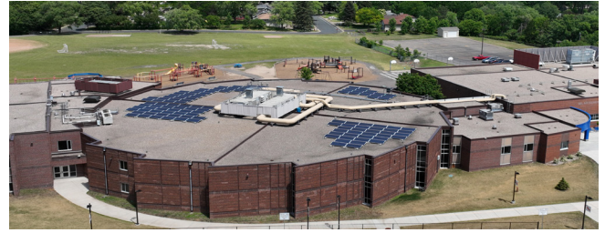
The solar array atop Bel Air Elementary School.
