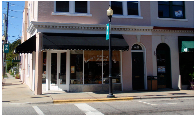
A SHOPFRONT WITH A CHAMFERED CORNER ENTRY.
