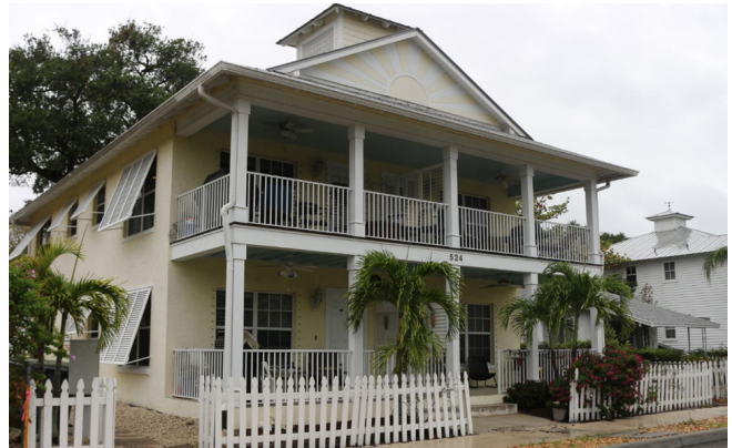
A 2-STORY PORCH ON AN APARTMENT BUILDING.
