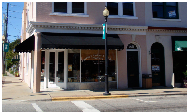
A SHOPFRONT WITH A CHAMFERED CORNER ENTRY.
