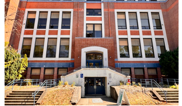
Current entrance to the JHS building by Kerby Ave.
