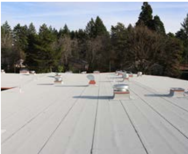
West Sylvan Middle School - New Roof, December 18, 2023
