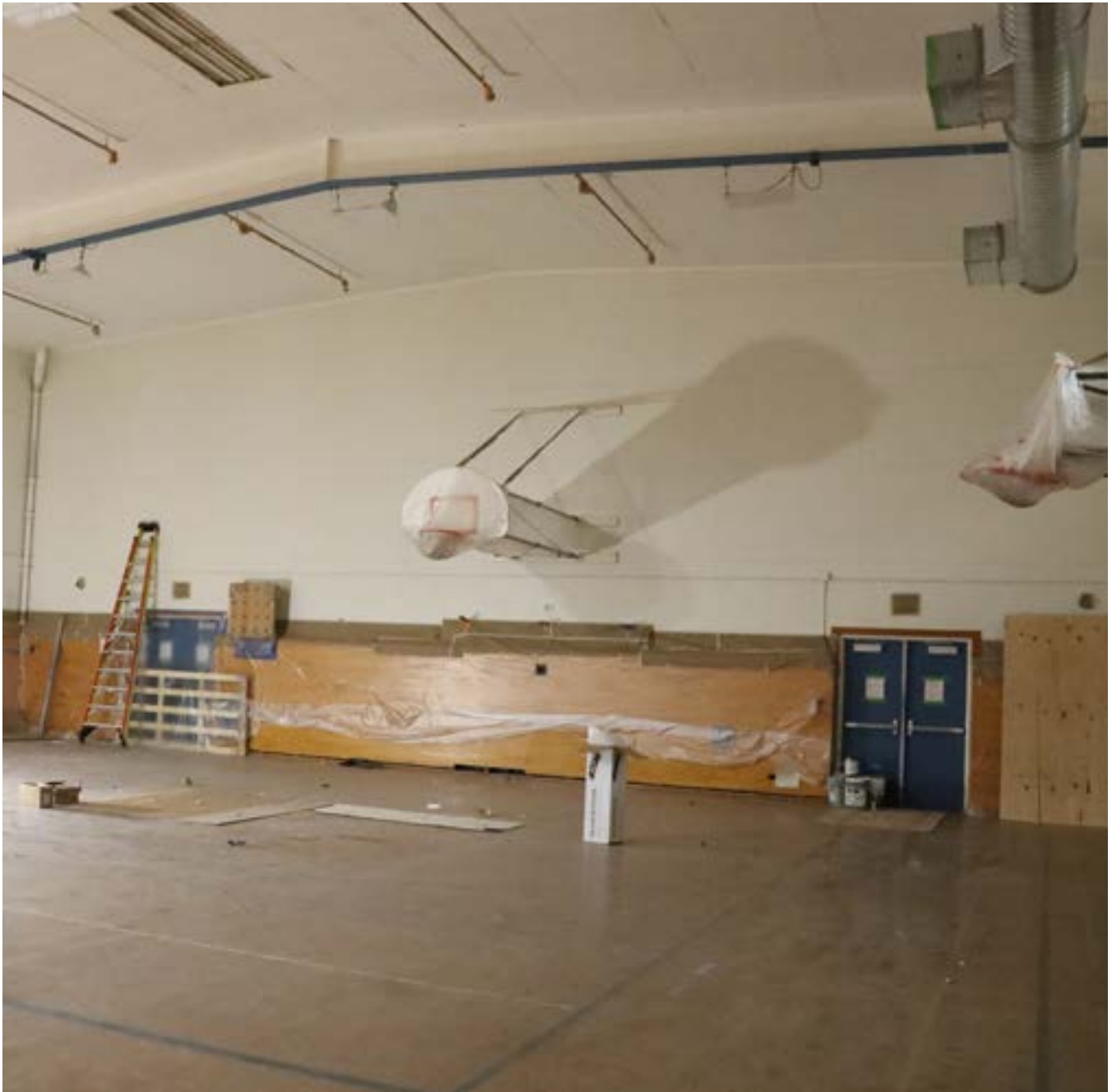
Harrison Park Middle School - Gym Construction, March 4, 2024
