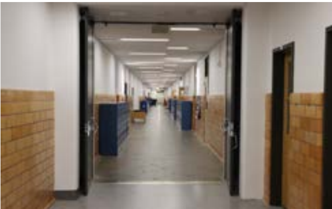
Harrison Park Middle School - Conversion Hallway, March 4, 2024
