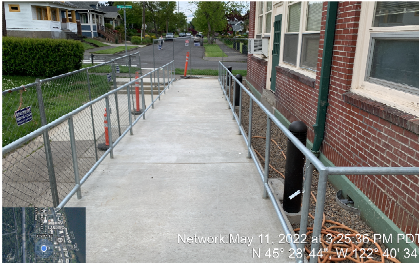
• New ADA ramp at Main Building entrance
