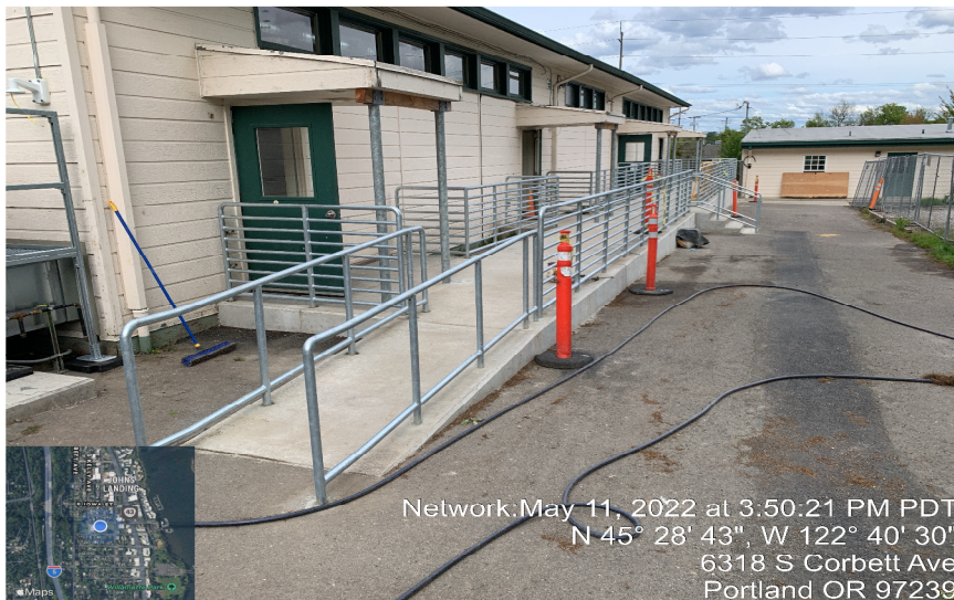
New ADA ramp at Modular 1 building
