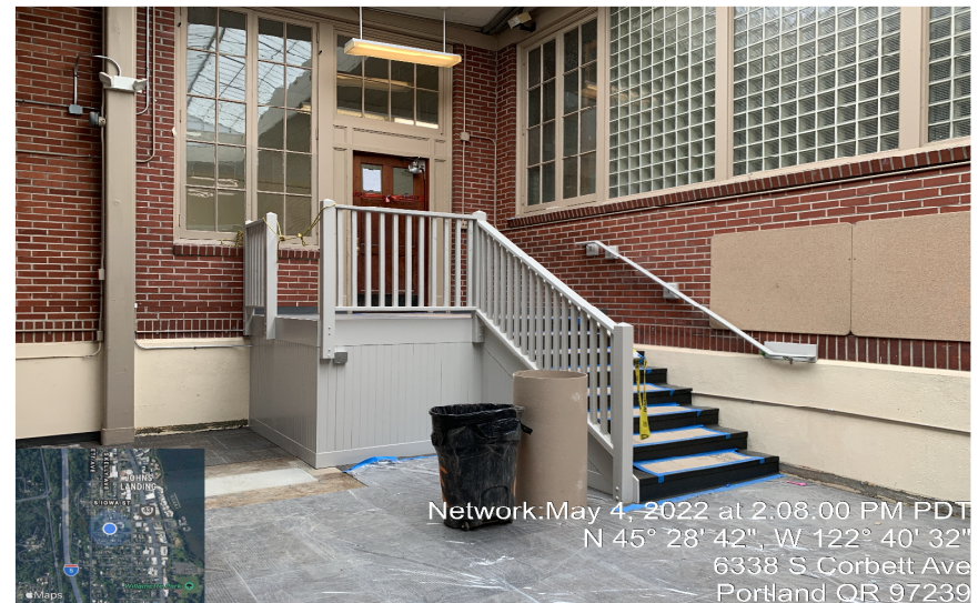
Updated landing and stairs in Main Building library
