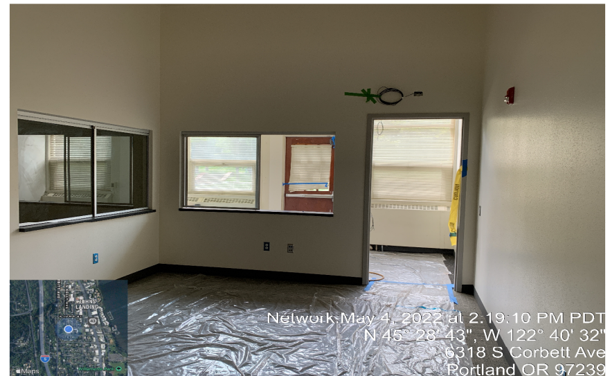
Construction of new admin suite in Main Building
