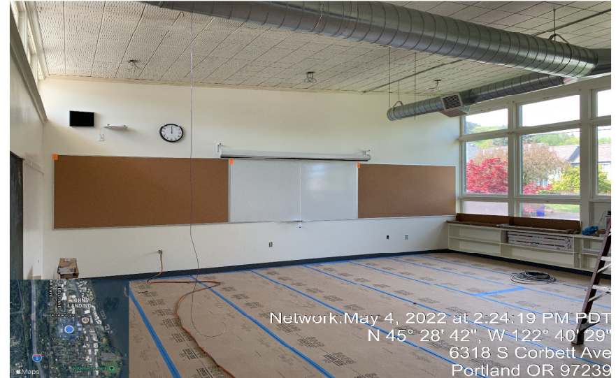
Teaching wall in Modular 1 classroom
