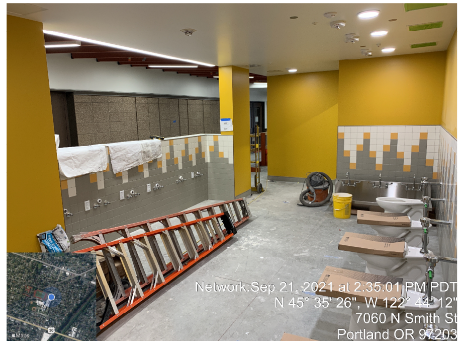
Build-out of RHS P4 addition all-user restroom.
