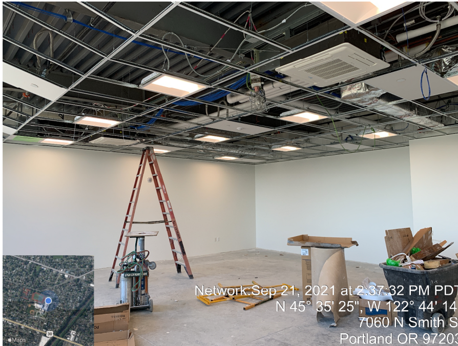
New classroom on 1 st floor of RHS P4 addition.
