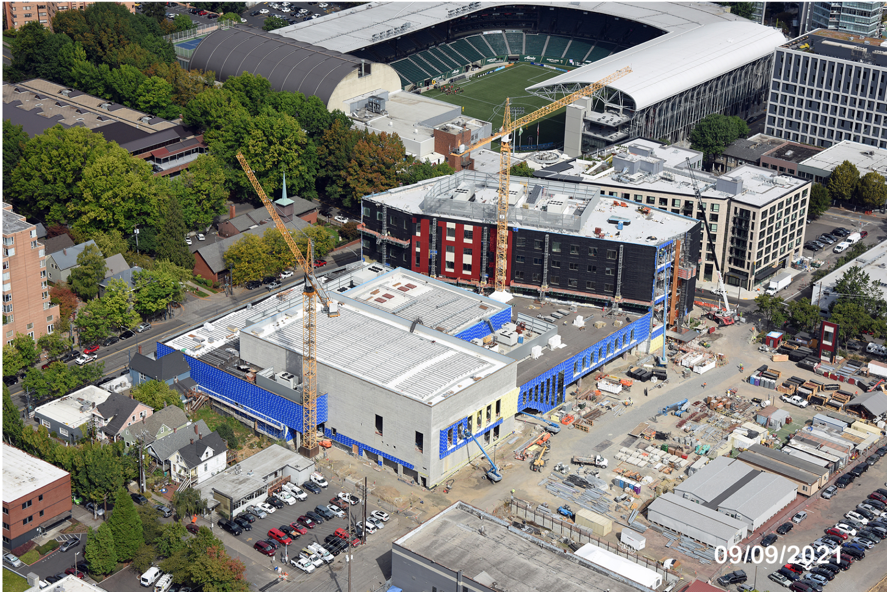
Aerial photo – September 9, 2021
