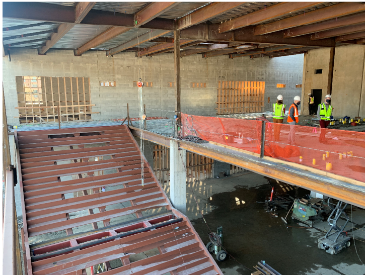
Steel stairs leading to the gym
