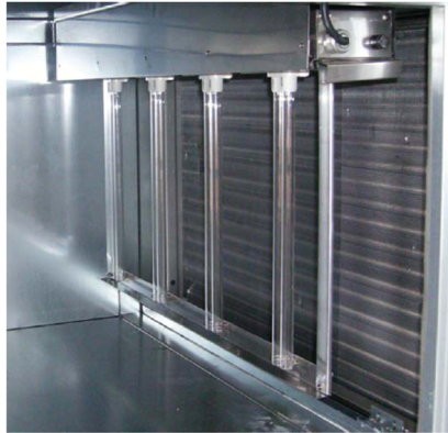
Typical in-duct UVGI installation with lamps mounted downstream of the cooling coil and drain pan
