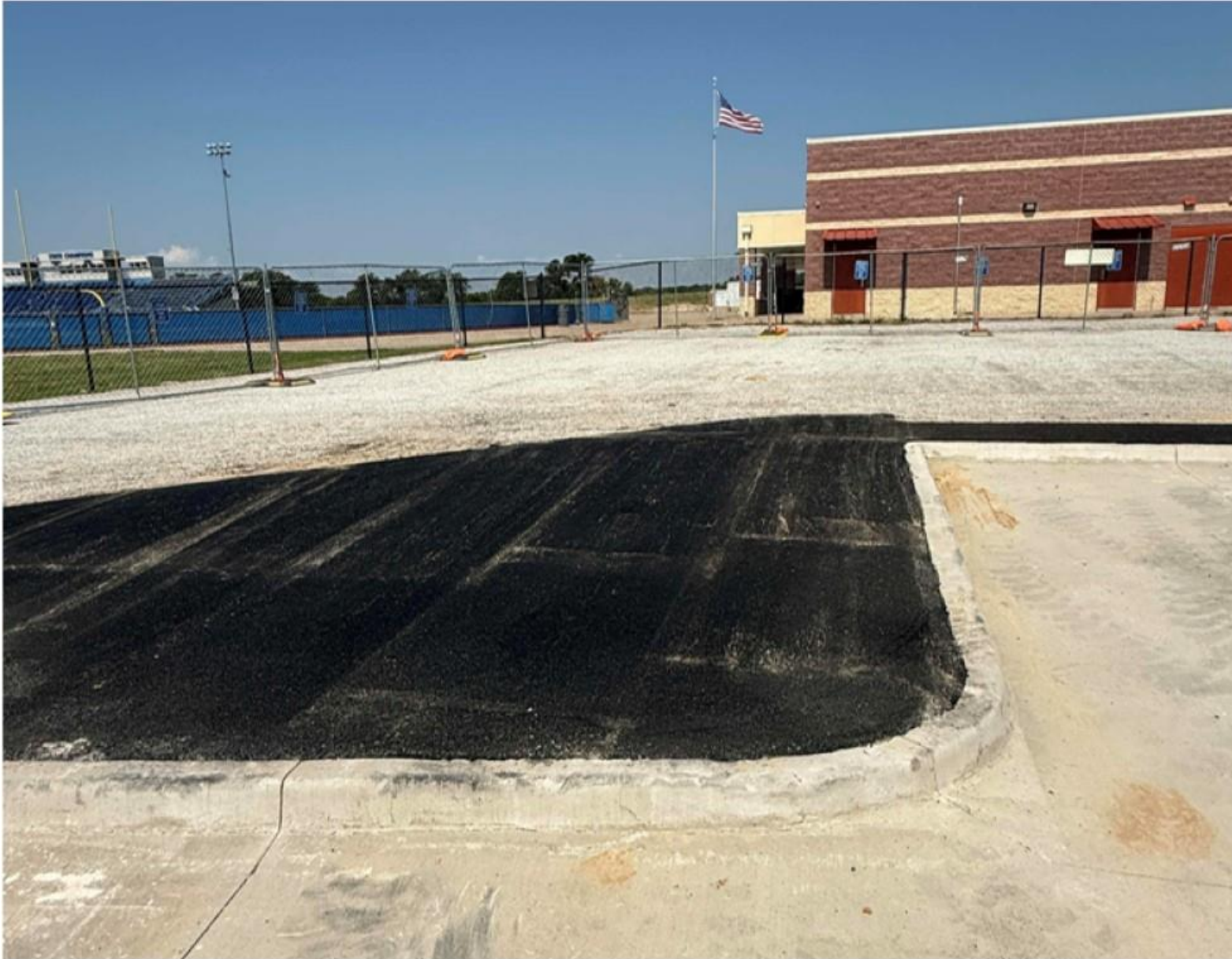
Asphalt Repairs on the West of Building
