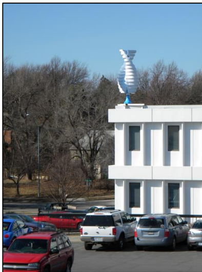
A Helix Wind Turbine on top of a Lincoln, Nebraska Office building.
