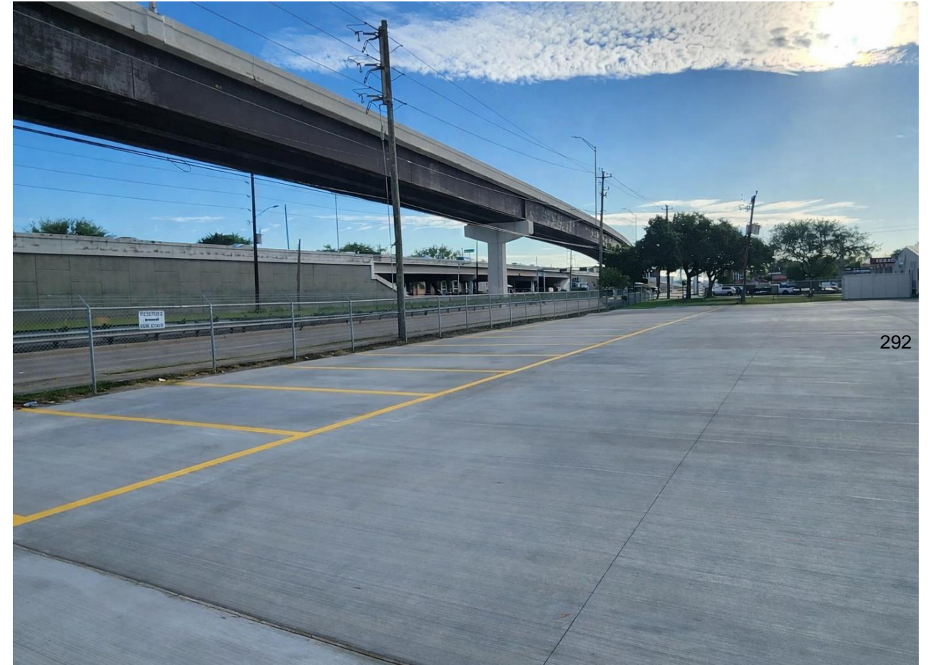
New concrete pavement with new yellow striping
