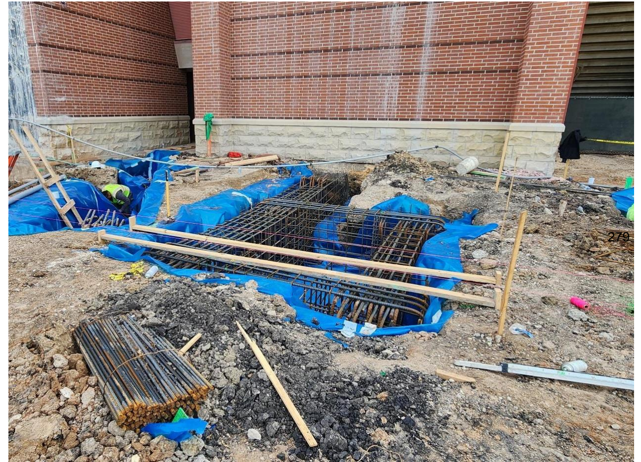
Grade beam steel cage at elevator pit
