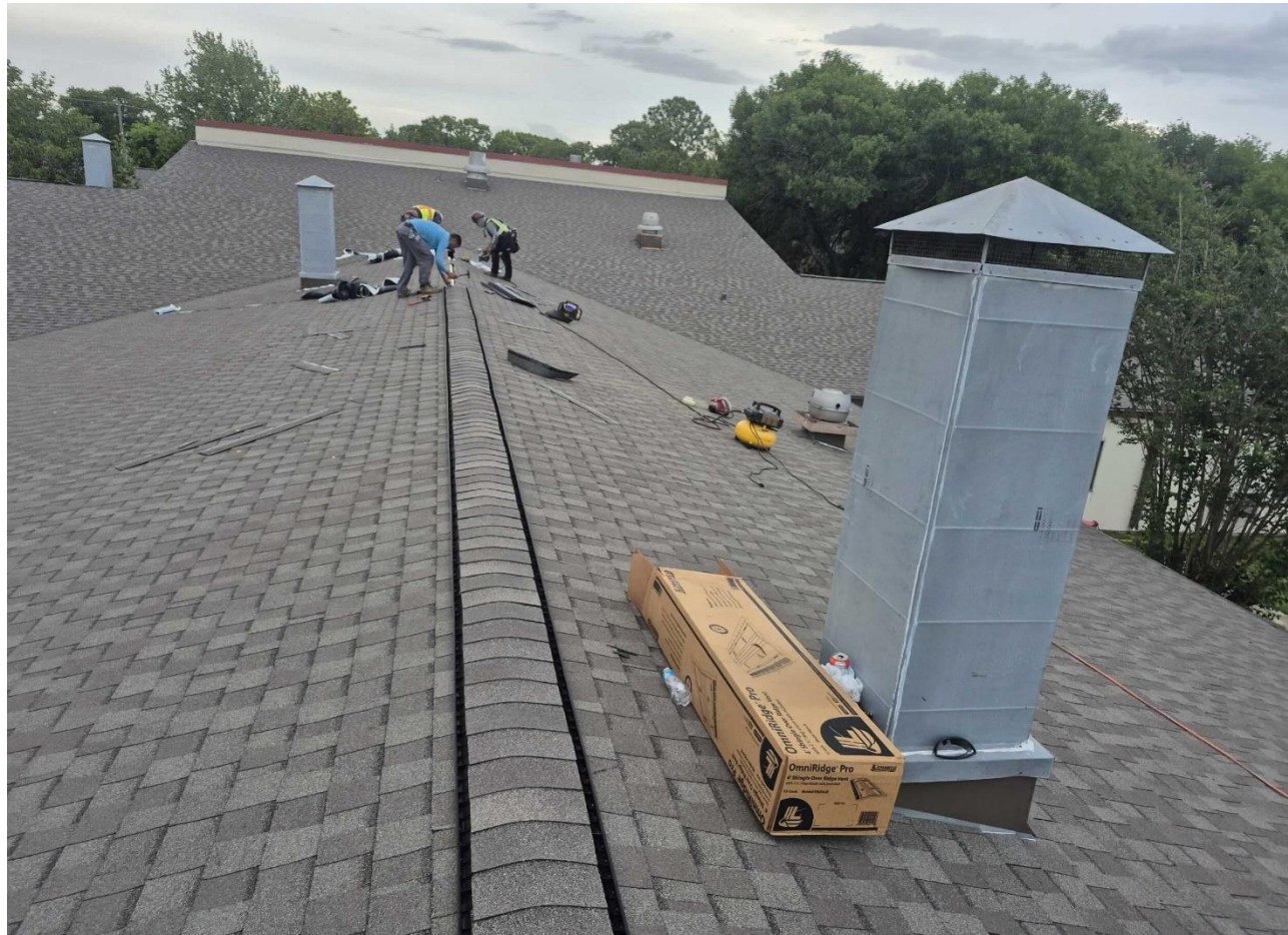
New shingle roof system replacement at Alief Learning Center
