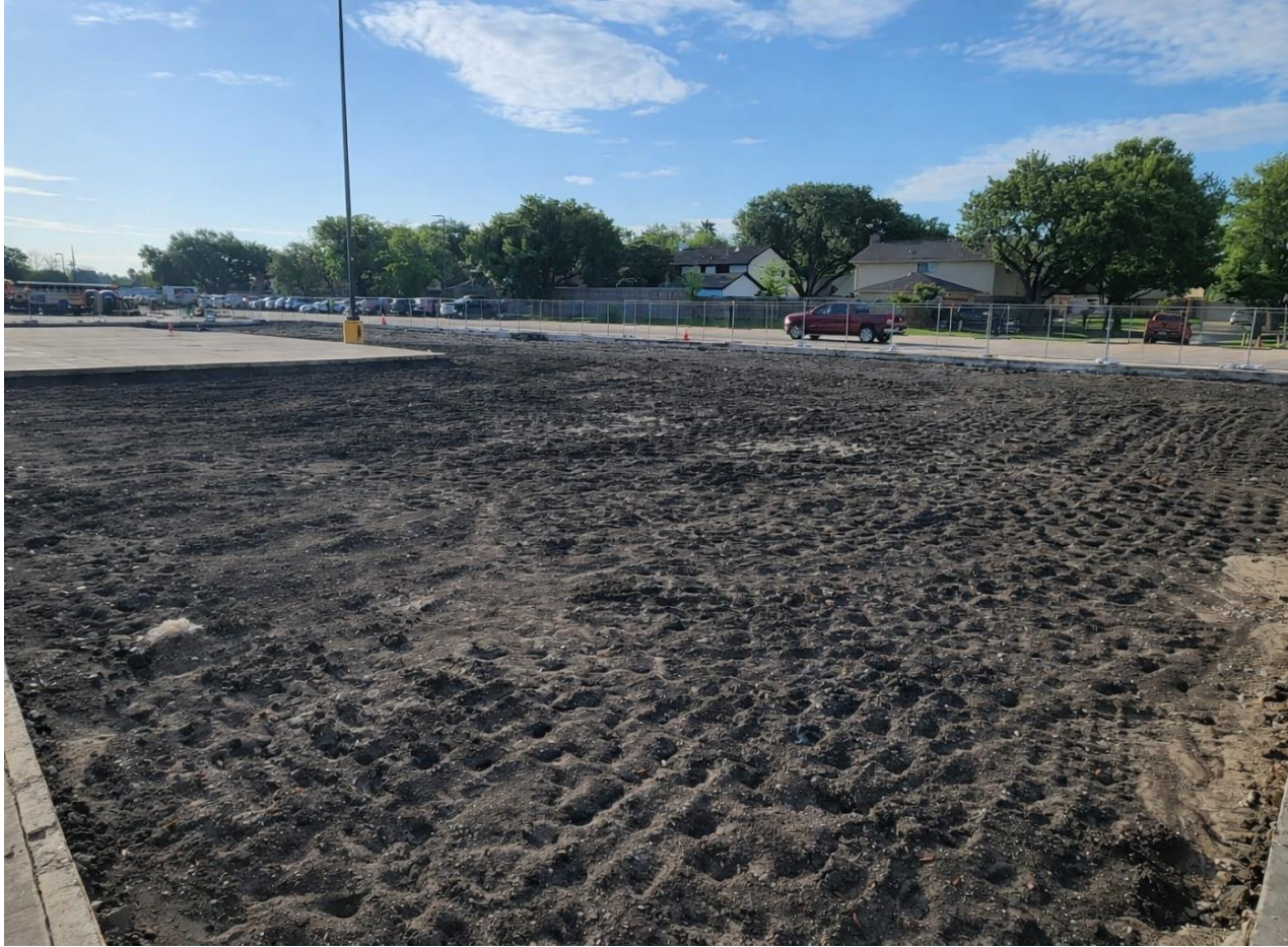
Concrete removal complete, soil compaction and rebar placement pending
