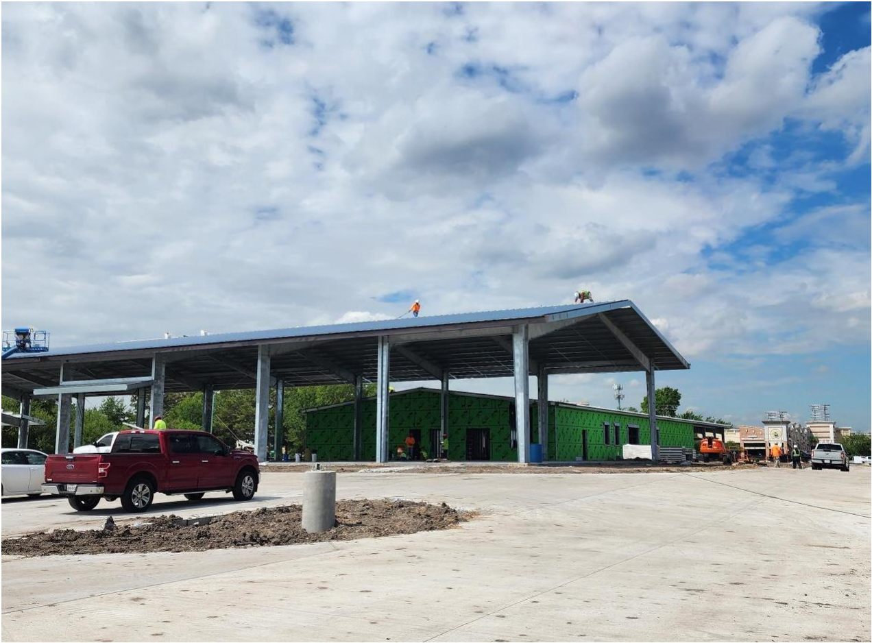
Structural detailing underway at the Show Arena
