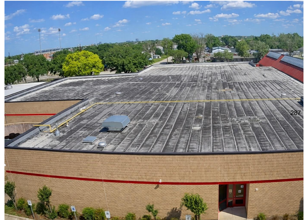
Base cover board installed at main building at Youens ES
