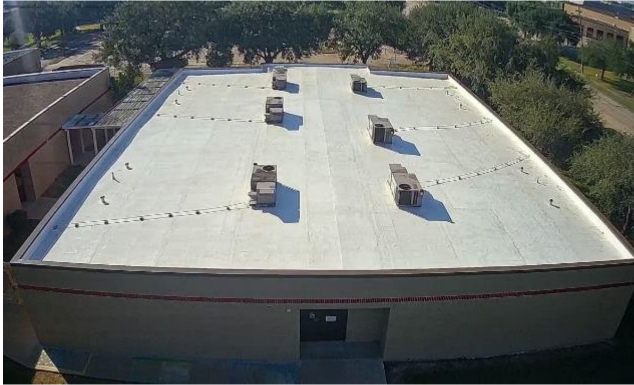
New Roof at Youens ES
