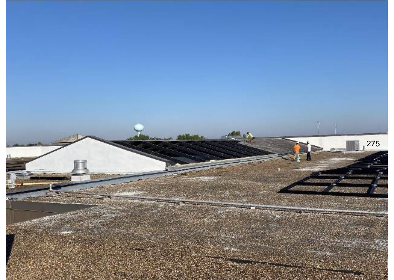
New Skylight Installation Underway at Elsik HS
