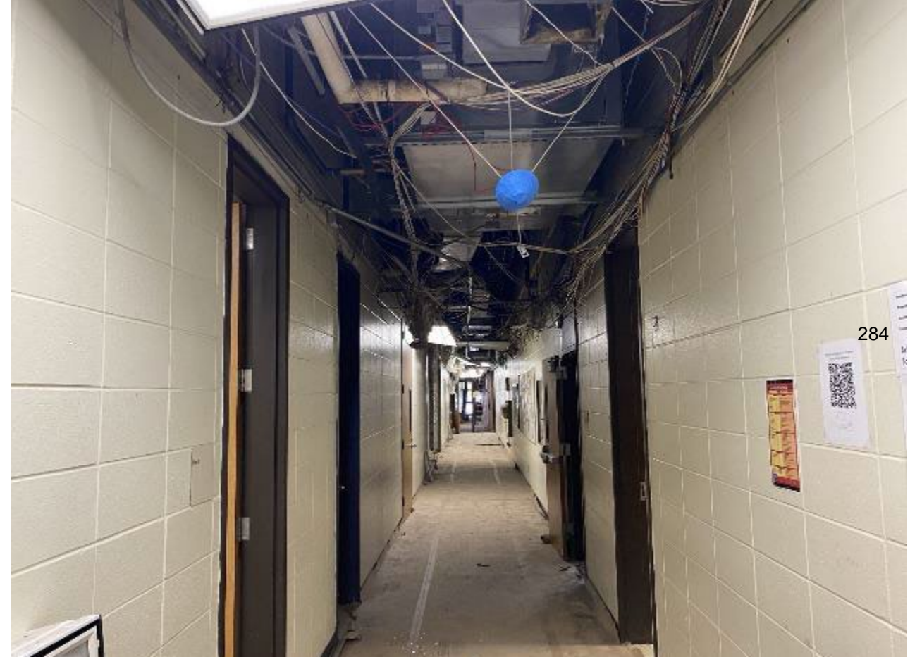
Mechanical Upgrades at Maintenance Bldg.
