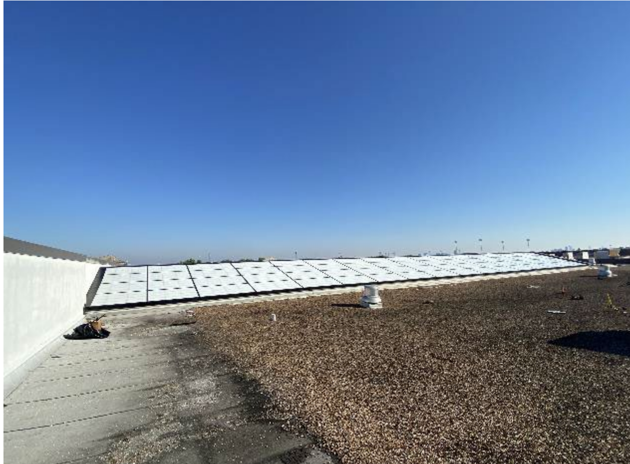
New Skylight System at Elsik HS
