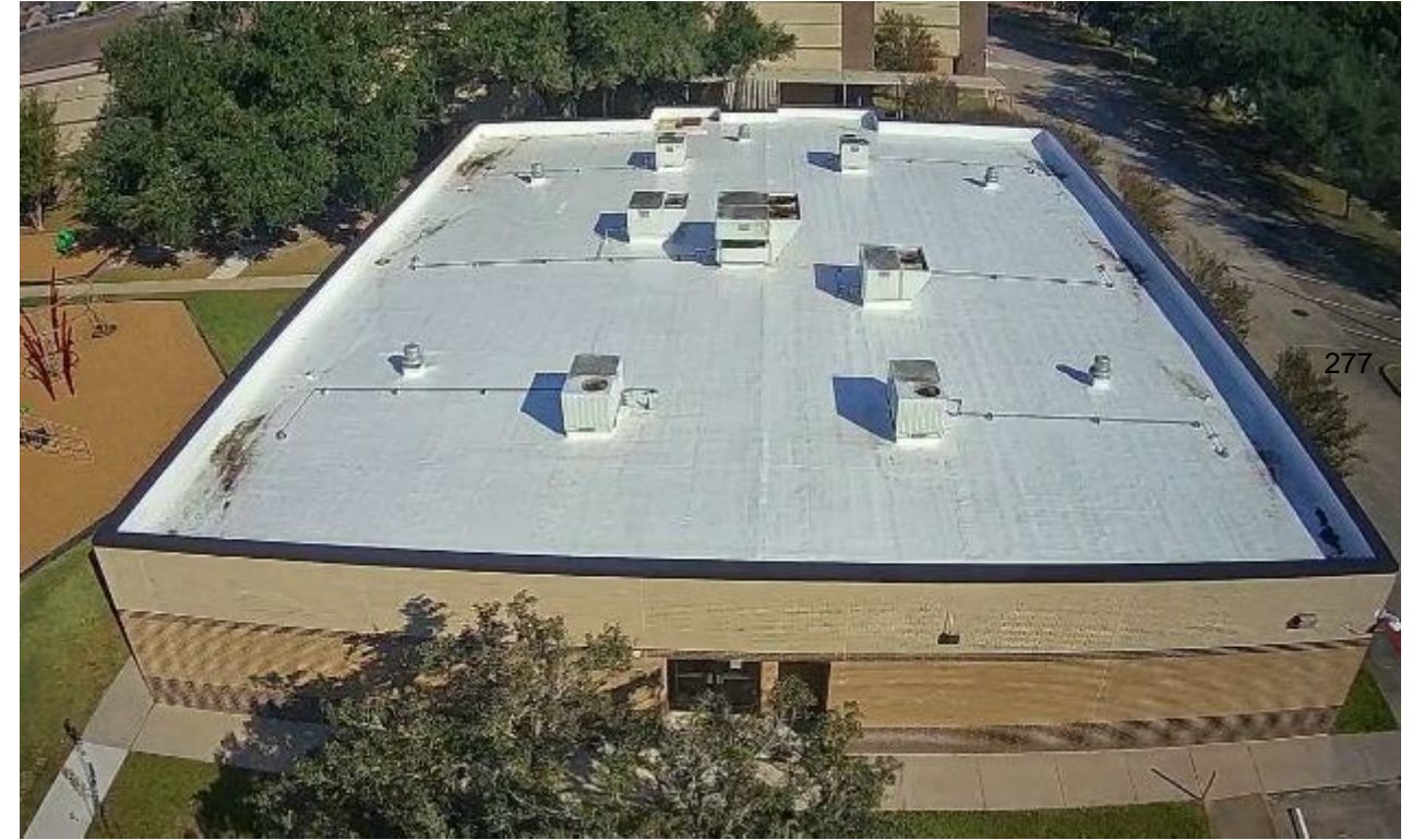
New Roof at Chancellor ES
