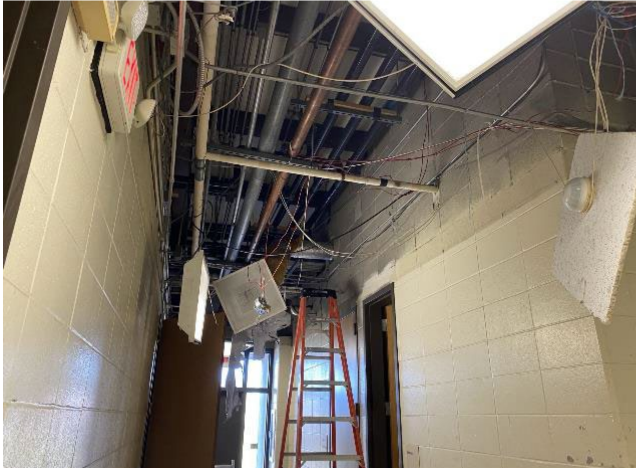
Mechanical Upgrades at Maintenance Bldg.
