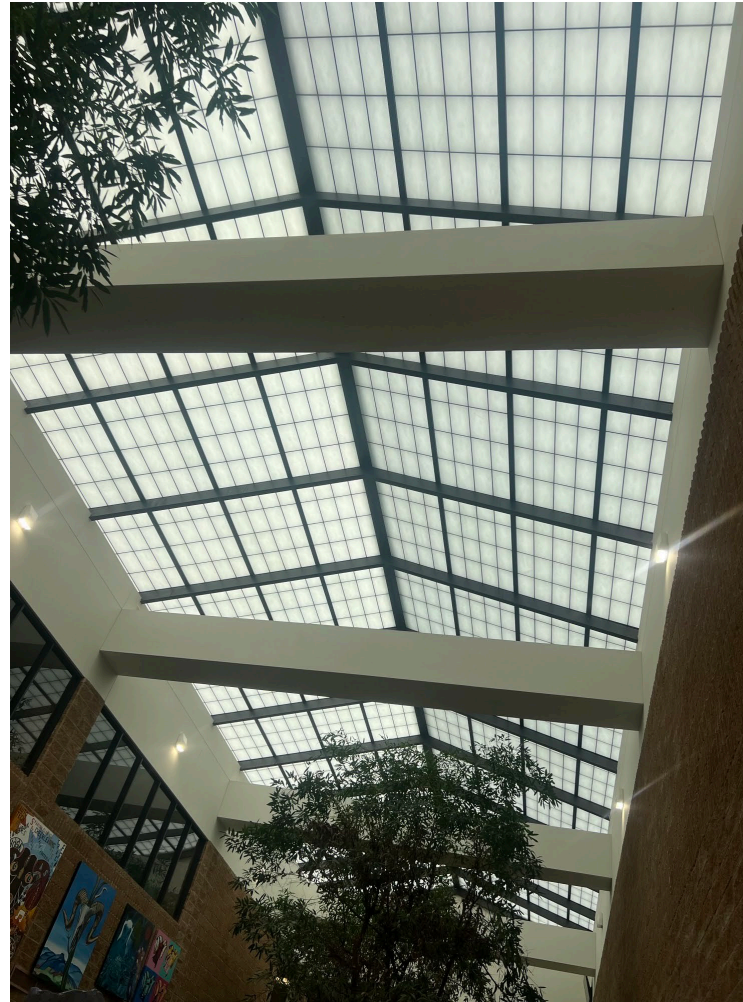
New Skylight System at Elsik HS
