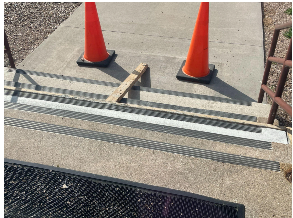
Repaired back step
