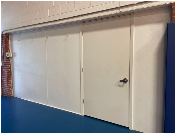
New gym interior wall
