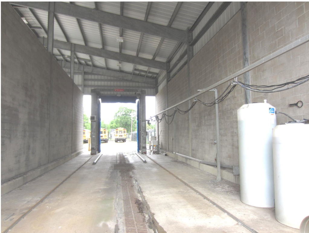
INTERIOR OF WASH BAY
