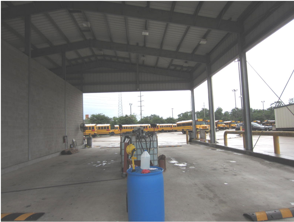
INTERIOR OF FUEL SHED
