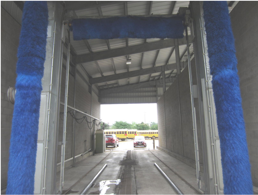
INTERIOR OF WASH BAY
