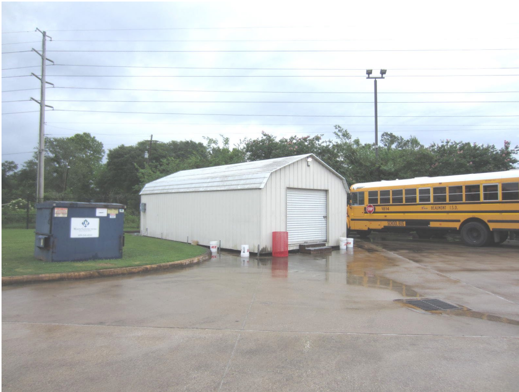
SOUTHWEST ELEVATION OF PORTABLE STORAGE BUILDING
