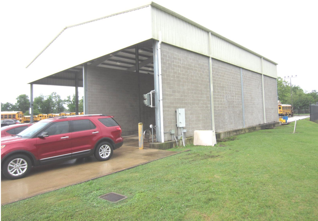
NORTHEAST ELEVATION OF WASH BAY/FUEL SHED BUILDING
