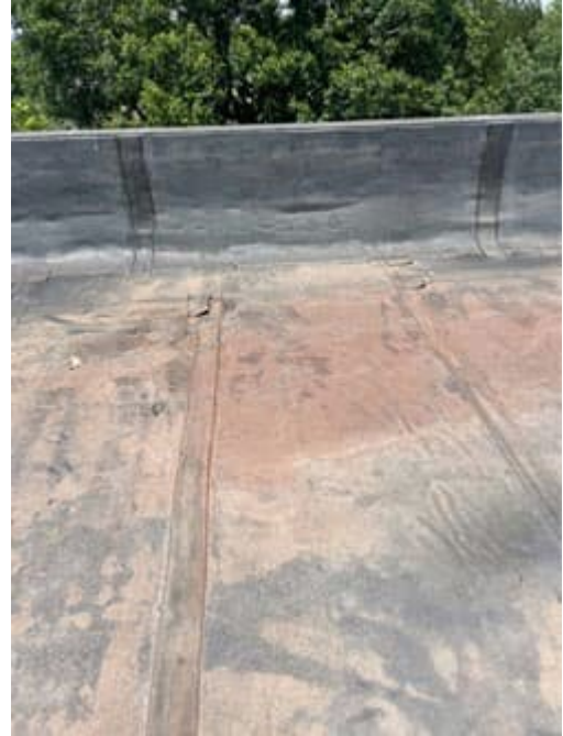
Ponding/shrinking
