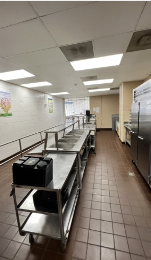
BP014 – Kitchen Renovations
