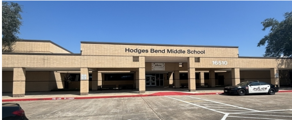
BP024 - Façade Upgrades & Renovations
