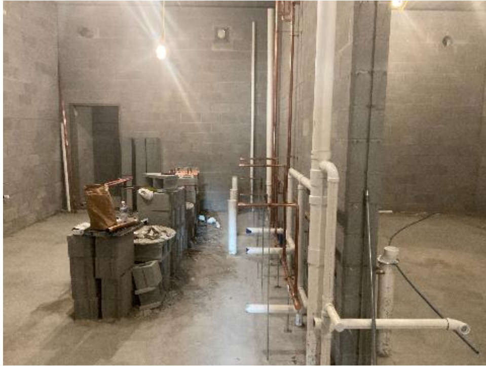
Restroom Plumbing Rough-In
