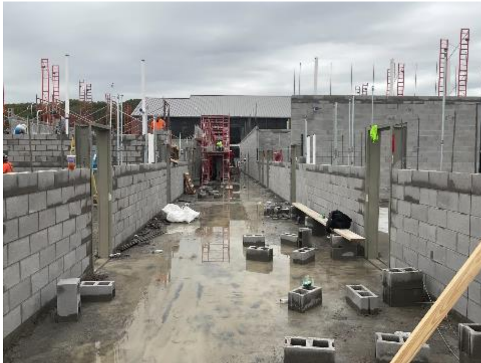
Second Floor CMU Installation
