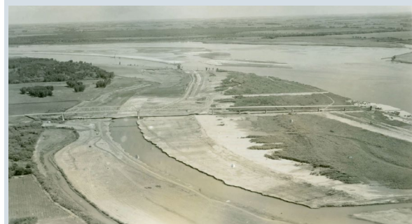
Photo: Partially completed bridge & USACE excavation, 1955.
