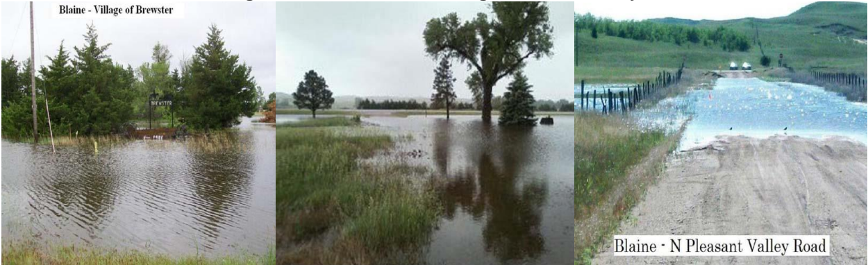
Figure 23: Localized Flooding in Blaine County
