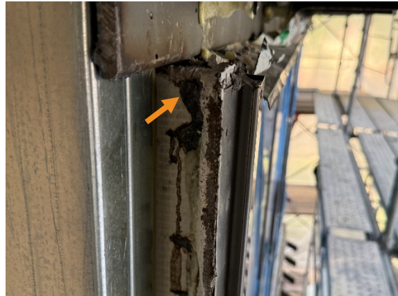
Figure 6. ArmorWall panel return at the jamb of the storefront window rough opening at the north elevation, similar to the jamb conditions at the west elevation. Note the black material on the backside of the ArmorWall sheathing (arrow).
