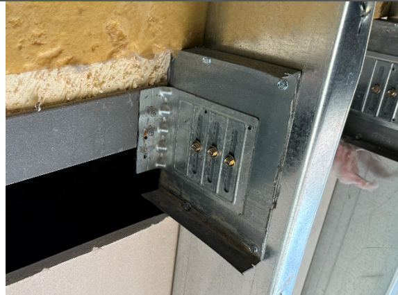
Figure 5. Clips attaching studs to structural steel framing at north elevation. Wallboard extensions will need to be notched around the clips.
