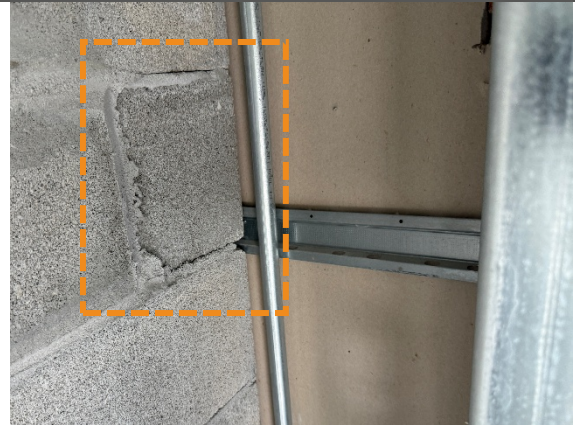
Figure 13. Rotated CMU at corner (orange box).
