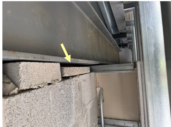
Figure 5. Gypsum board to be notched and fit tightly to steel beam. Voids in between beam and CMU to be filled prior to SPF installation (arrow).
