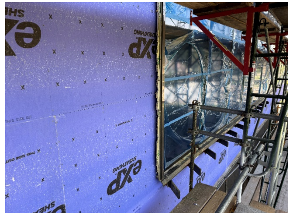
Figure 15. View of Type X sheathing installed at west elevation.
