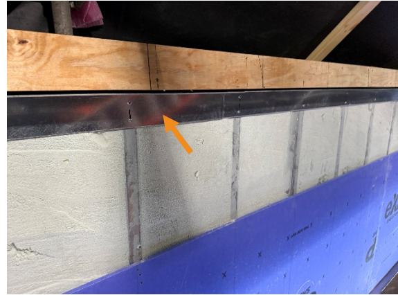
Figure 16. Bent plate installation at west parapet. Note that the sheathing was temporarily removed to allow for bent plate installation.
