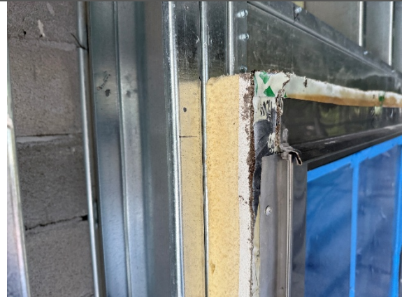
Figure 8. Punched window jamb at CMU backup. Based on initially exposed conditions, it is not clear if there is an ArmorWall sheathing return at the jamb.
