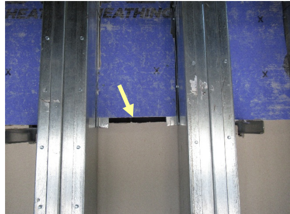
Figure 7. New wallboard extensions. All gaps/voids to be sealed prior to installation of SPF (arrow).
