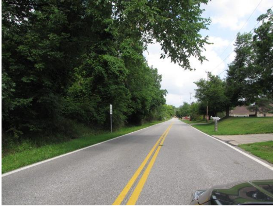
W. Mill Road; North
