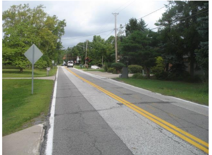
W. Mill Road; north
