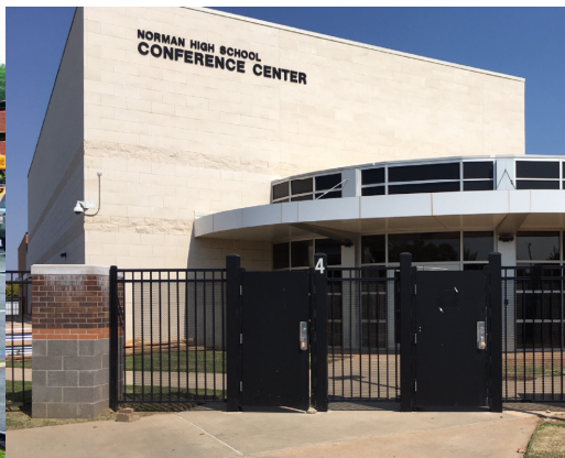
OPTION 1: 6' ORNAMENTAL FENCE WITH 2 GATES (APPROX. 880 LINEAR FEET). NEW GATES CAN BE ACCESSED FROM THE OUTSIDE BY THE FIRE DEPARTMENT AND TEACHERS WITH ELECTRONIC LOCKS. (SAMPLE IMAGES)
