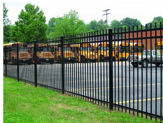
OPTION 1: 6' ORNAMENTAL FENCE WITH 2 GATES (APPROX. 880 LINEAR FEET). NEW GATES CAN BE ACCESSED FROM THE OUTSIDE BY THE FIRE DEPARTMENT AND TEACHERS WITH ELECTRONIC LOCKS. (SAMPLE IMAGES)
