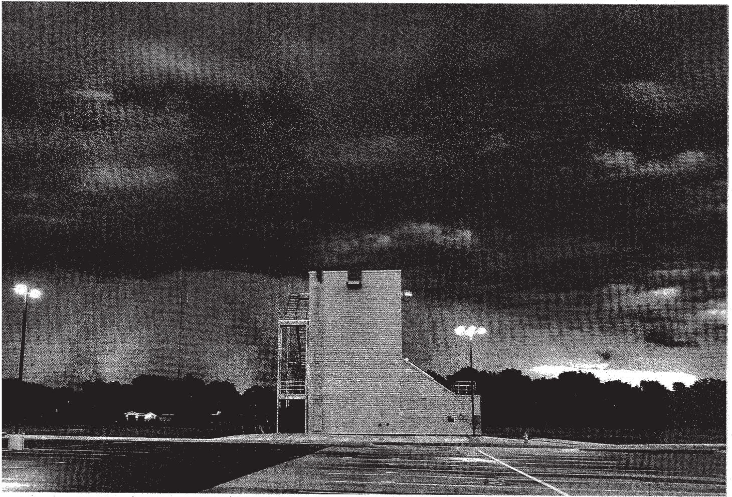
City's new Emergency Services Training Center, completed in August will benefit not only the full-time career programs, but also education for industry. The tower stands 44 feet high with 18,425 square feet of usable training space, including burn rooms and classrooms.
