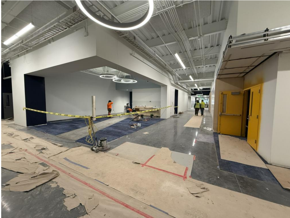
COMMON AREA HALLWAY | FIRST FLOOR
