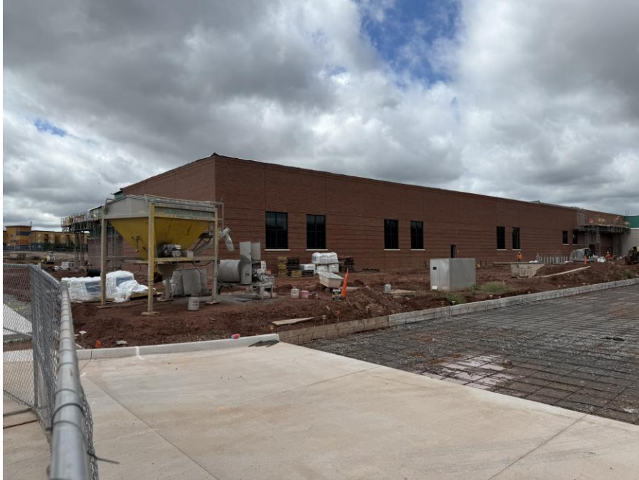
AREA 6 – PA WING SE EXTERIOR
