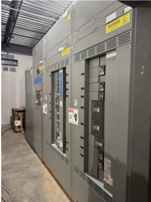
AREA 5 – ELECTRICAL ROOM BUILD OUT
