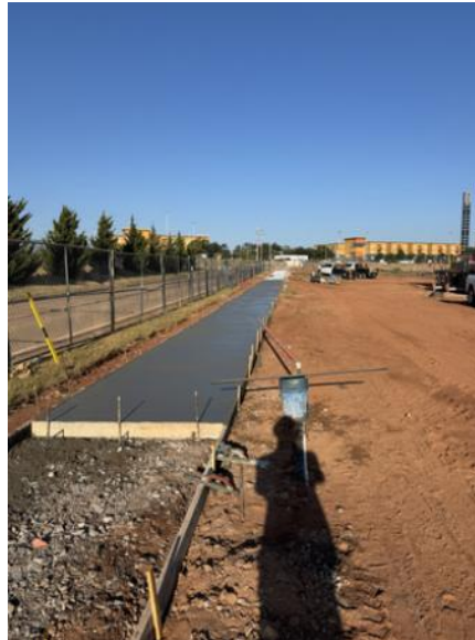
SITE – SIDEWALK ALONG FRANKLIN
