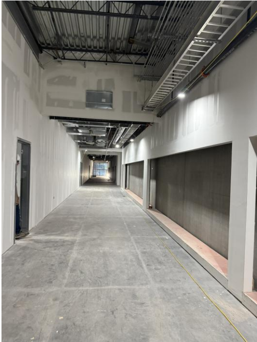
AREA 2 – 1 ST FLOOR SPED HALLWAY
