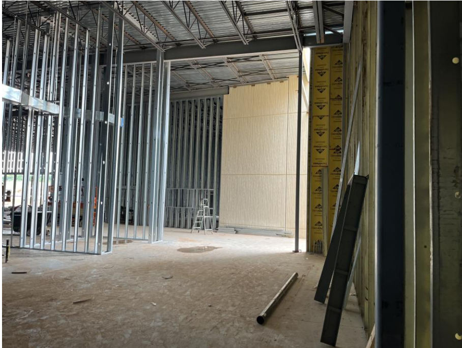
AREA 6 – PA WING COMMON SPACE FRAMING
