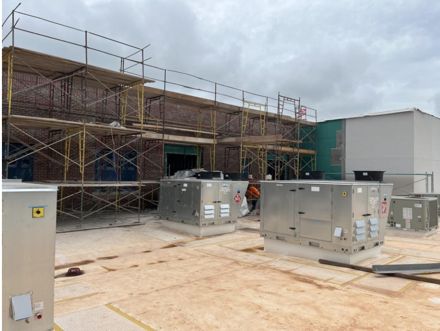
AREA 5 – EXTERIOR BRICK EAST SIDE
