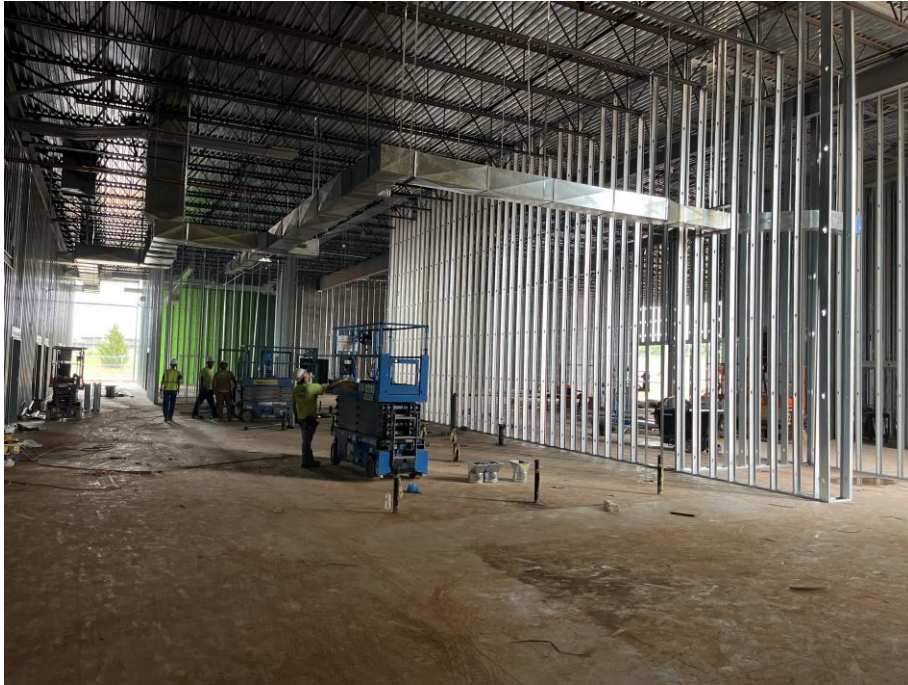
AREA 6 – PA WING INTERIOR METAL STUD FRAMING AND MEP ROUGH-IN
