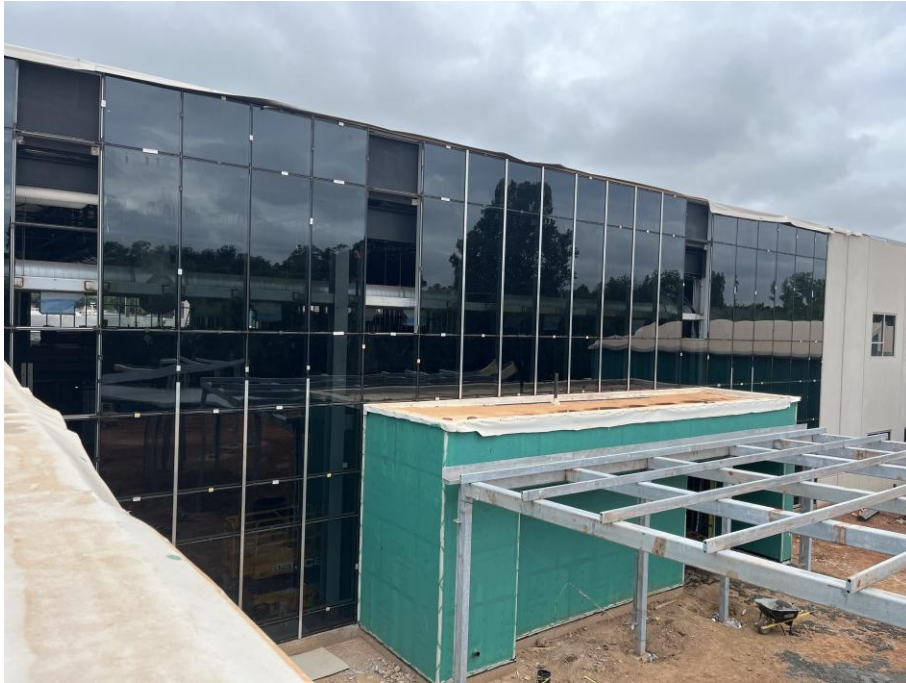
AREA 4 – STUDENT CENTER CURTAINWALL
