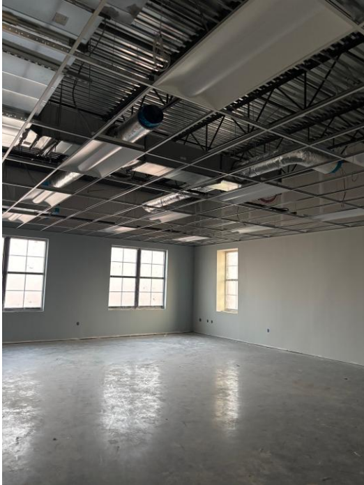
AREA 1 – CLASSROOM CEILING GRID AND LIGHTING
