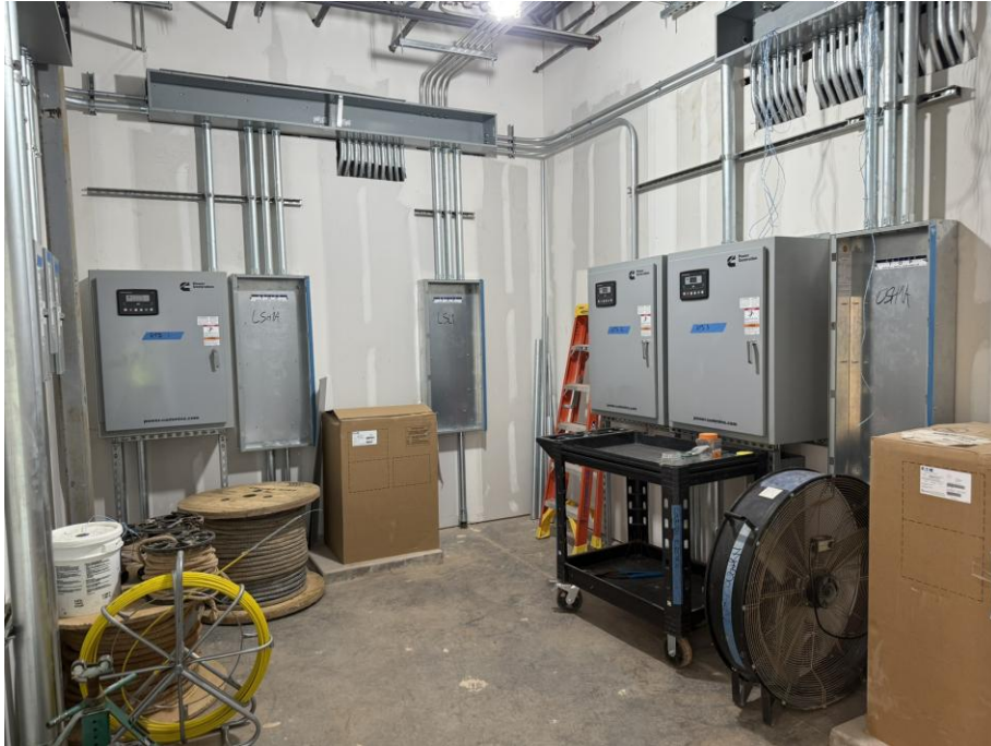
AREA 5 – ELECTRICAL ROOM BUILD OUT
