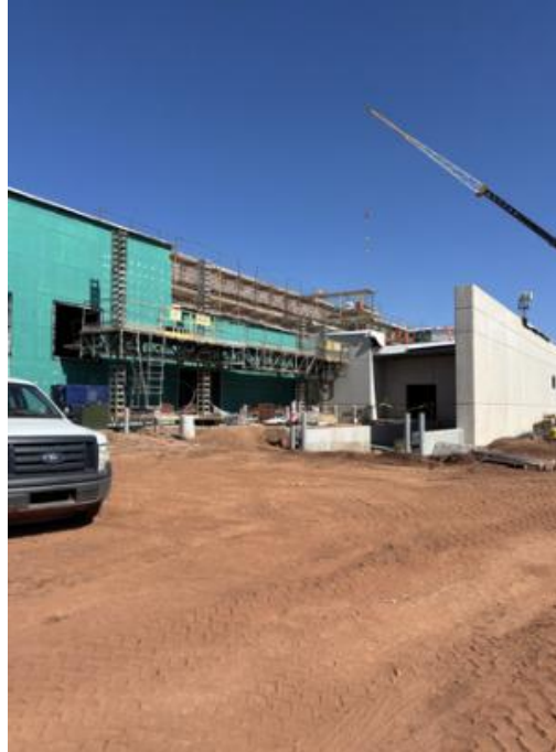
AREA 5 – LOADING DOCK BRICKWORK
