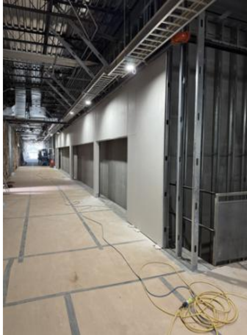
AREA 2 – LOCKER ALCOVES
