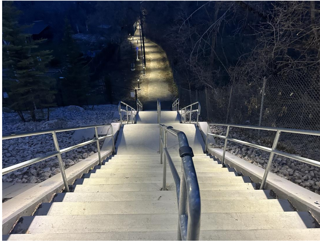
Stairway into the gully
