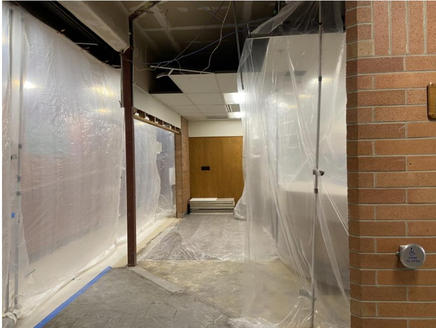
Demolition complete with dust barrier in place
