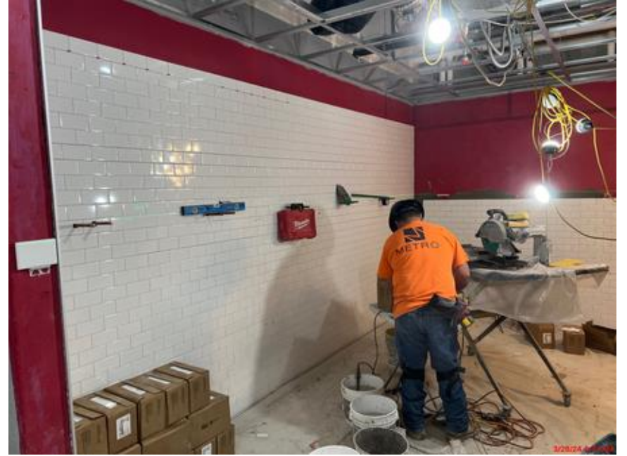
Tile in Pool Locker Room
