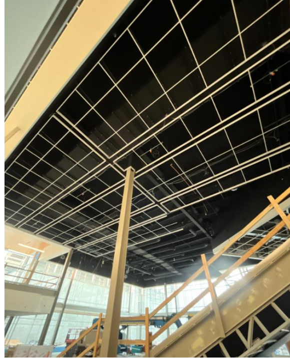
High ceiling clouds being installed in the Cafeteria
