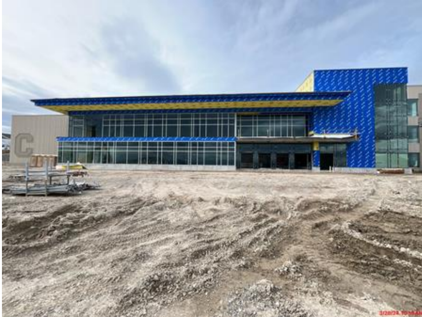
Curtain wall and glass installation on the exterior of the Auditorium 238
