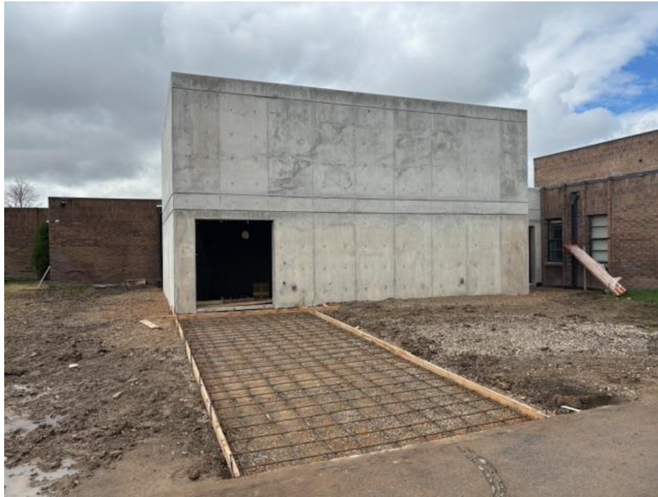
Central plant enclosure 227 nearly complete
