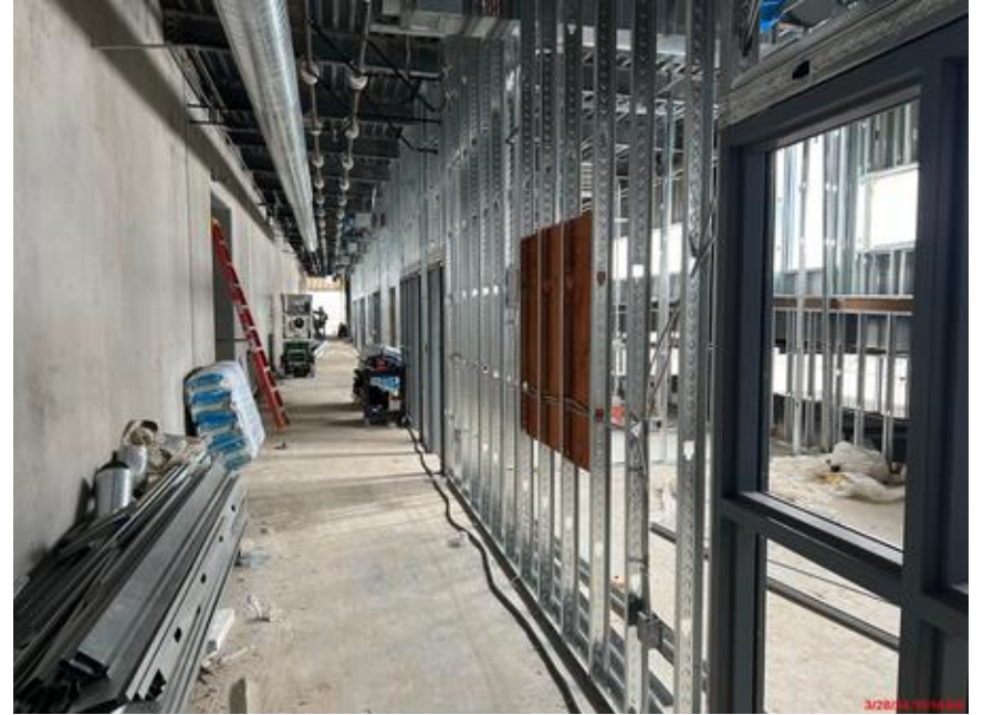
Framing and electrical in Administration Level 3
