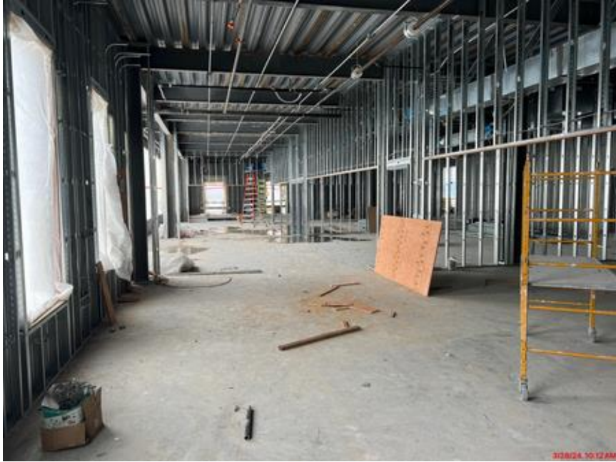
Framing in Administration Level 2
