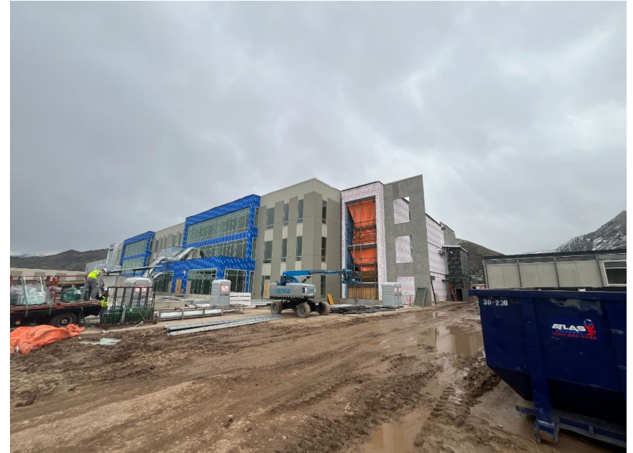
Stair tower connecting Academics to Performing Arts
