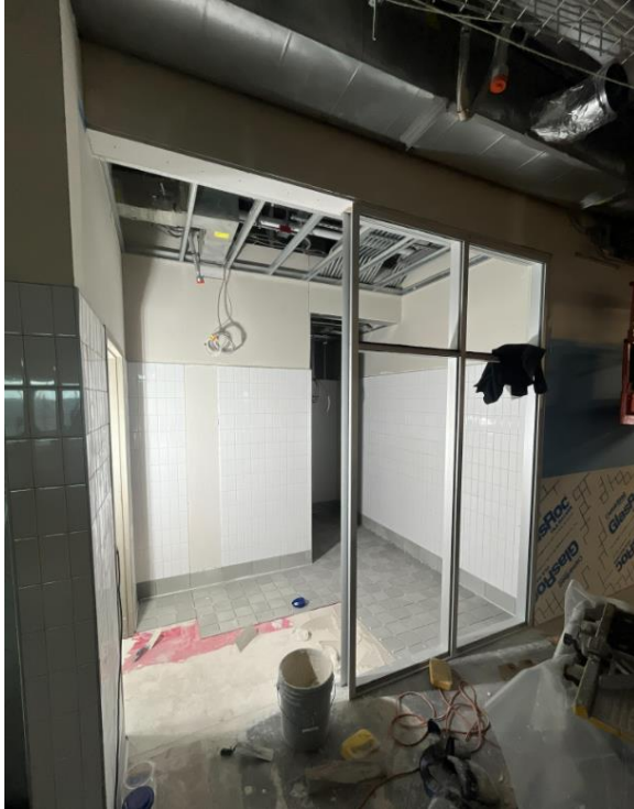
Tile and storefront being installed in Level 1 restroom
