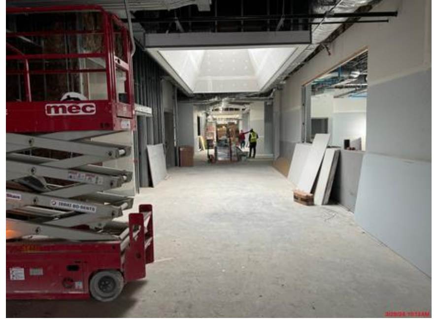
Drywall on Level 3 of classrooms in Academics
