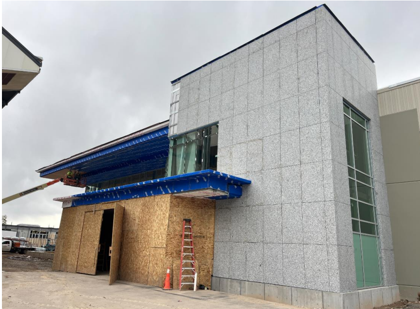
Stone cladding at the Main Entrance
