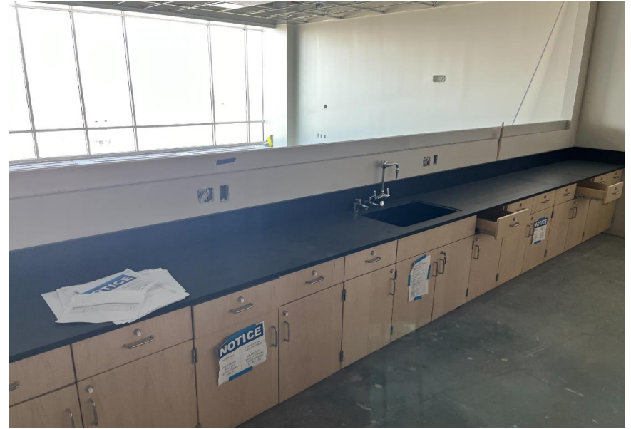
Countertops installed in Level 3 science labs
