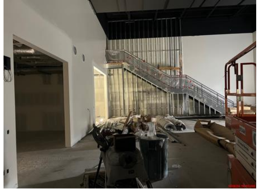
Paint and framing in the Scenery Shop
