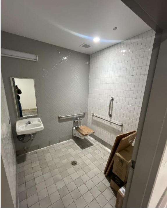
Plumbing fixtures and accessories installed in Administration Suite restroom
