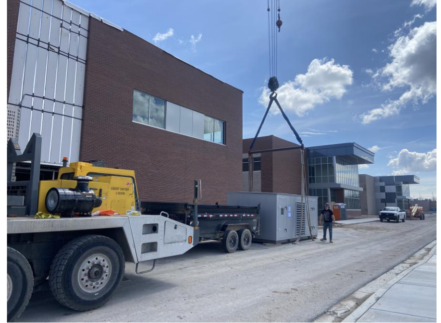
Delivery of air handling units
