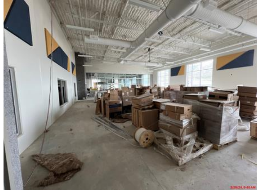
Tectum panels in the Weight Room
