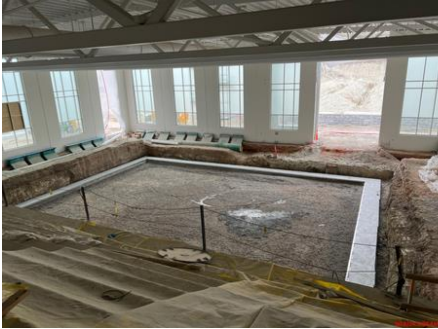
Pool excavated and footings poured
