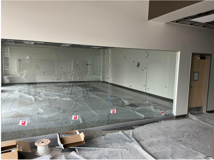
Glass installed at the Level 2 classrooms
