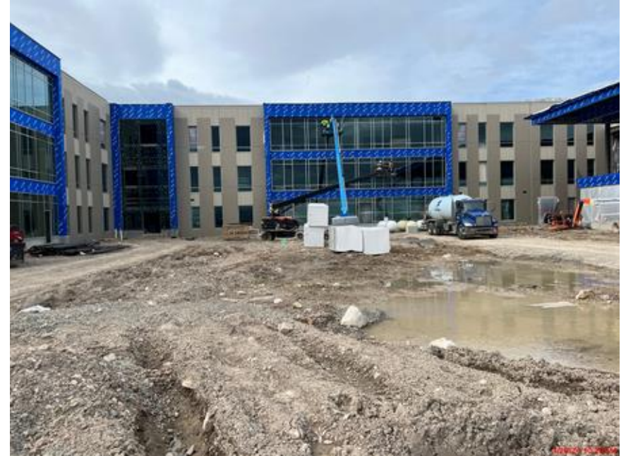
Curtain wall and glass installation on the exterior of Academics
