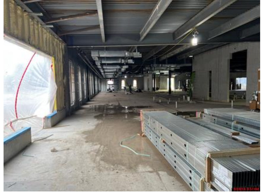
Framing and HVAC in Administration Level 1
