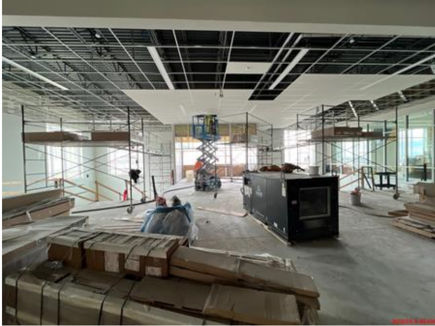
Ceiling tile in the Athletics Vestibule
