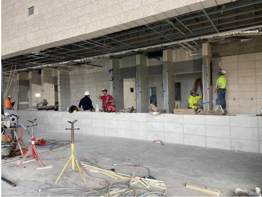
Tile work in Kitchen and Serving Areas
