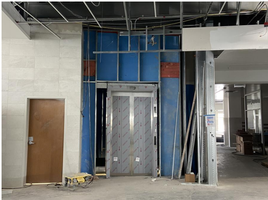
Elevator installation in progress
