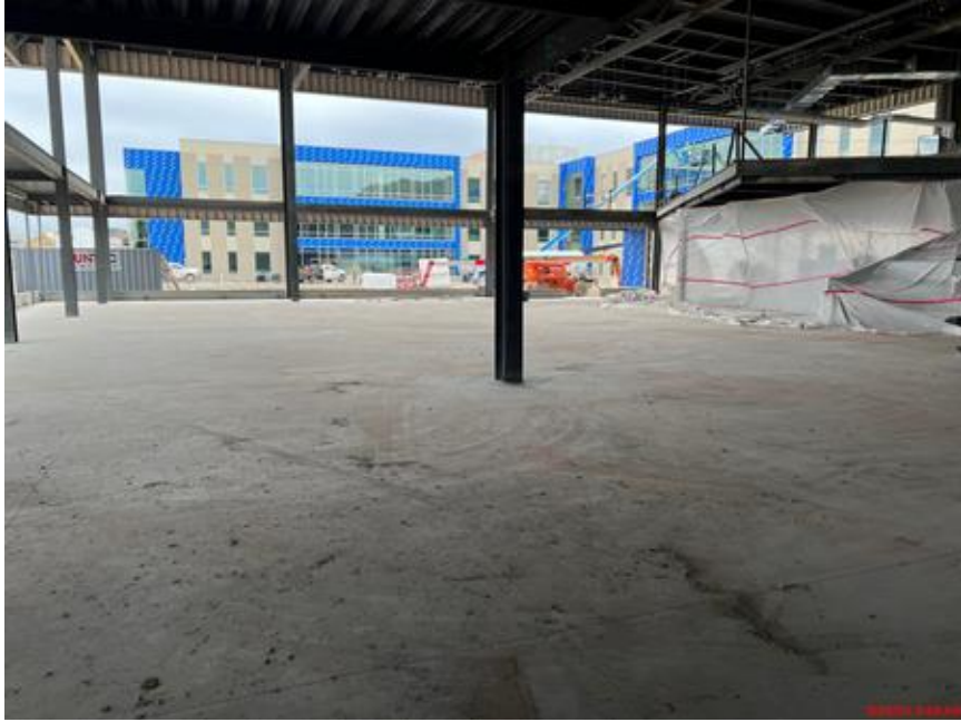
Slab on grade in Student Commons
