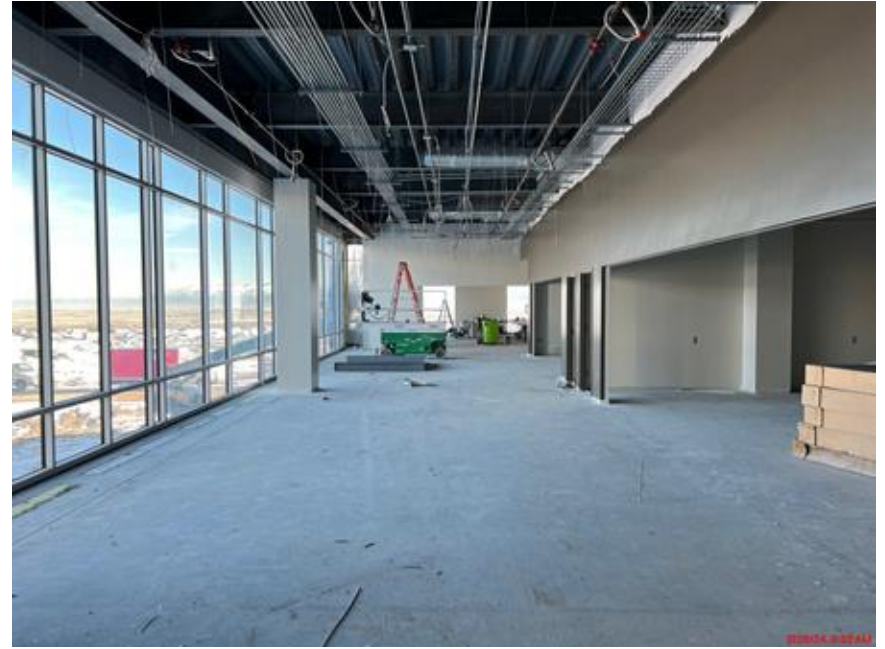
Paint on Level 2 of the Social Studies wing
