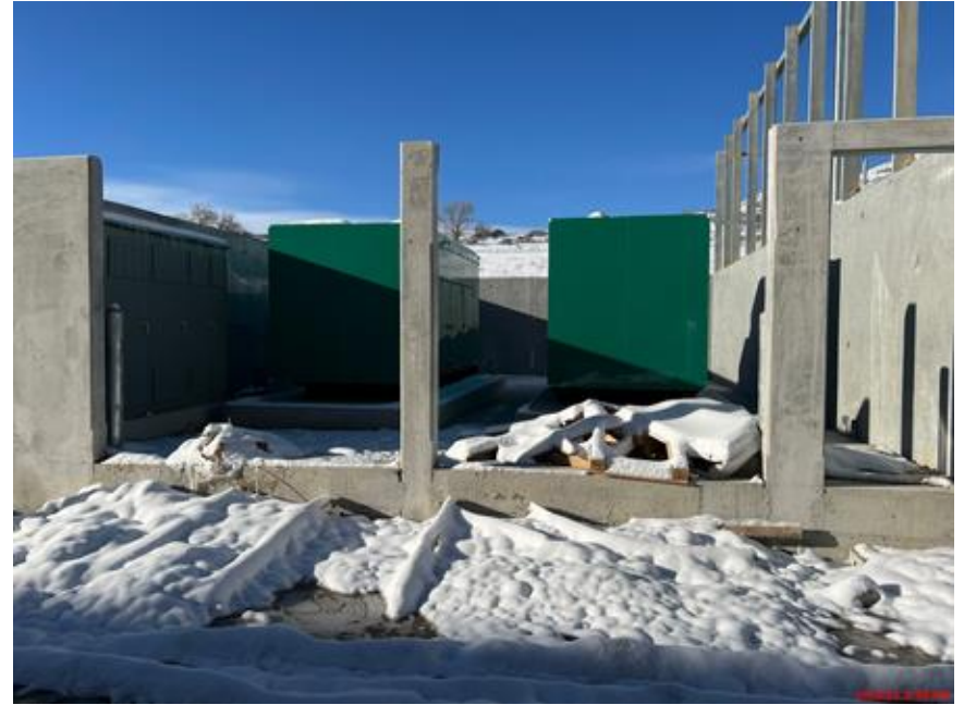
Setting the generators into place
