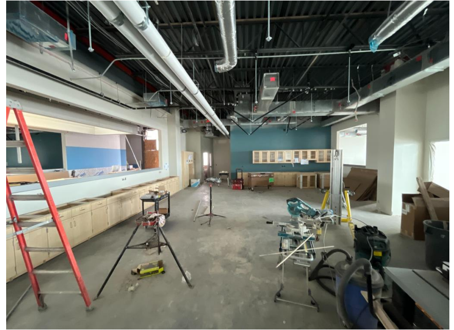
Cabinets installed in Level 3 Science classrooms
