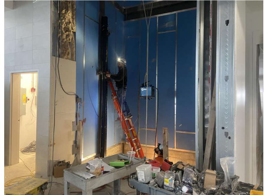
South elevator installation in progress
