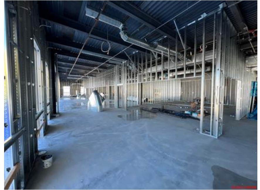
Framing on Level 3 of the Administration Building
