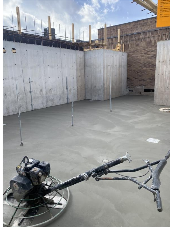
Concrete being finished
