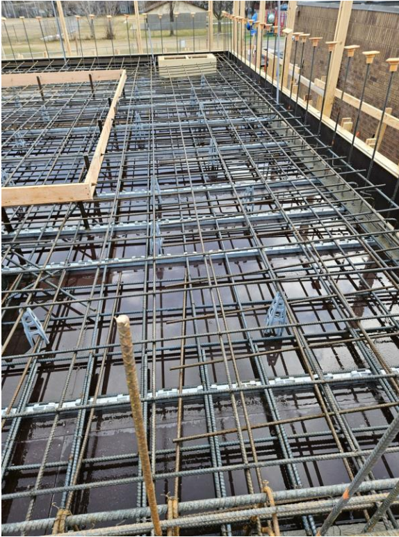
Rebar in place and ready for concrete
