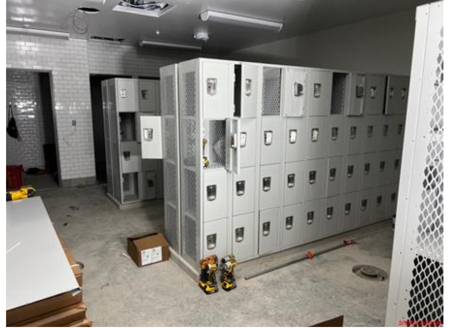
Lockers being placed in the PE Locker Room
