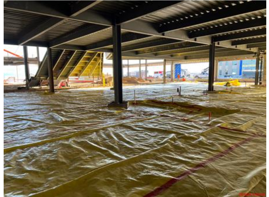
Prepping slab on grade in the Public Square/ Dinning Area
