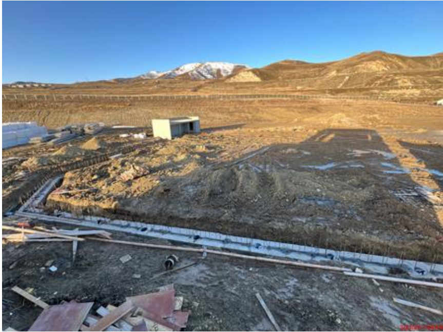
Softball Field footings/foundation
