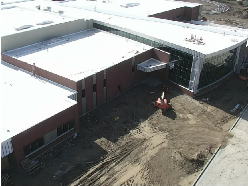
Glazing at North Entry
