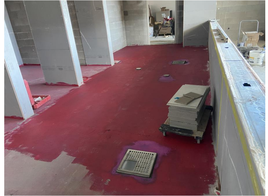
Preparation for floor tile in Kitchen
