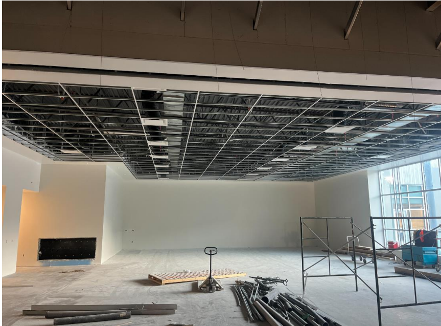
Ceiling grid in the Testing Center
