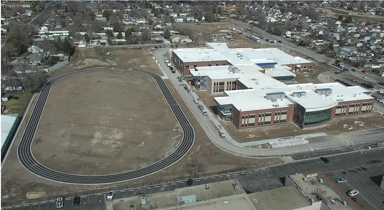
South view of project site
