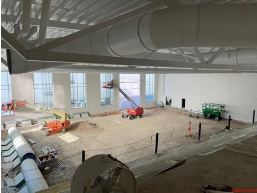
Pool painting and window caulking
