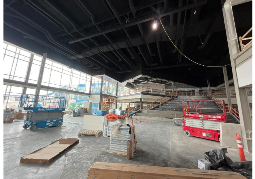
Exterior glass and painted ceiling in Cafeteria/Commons
