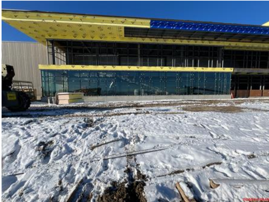
Curtain wall and glazing around the Auditorium Lobby
