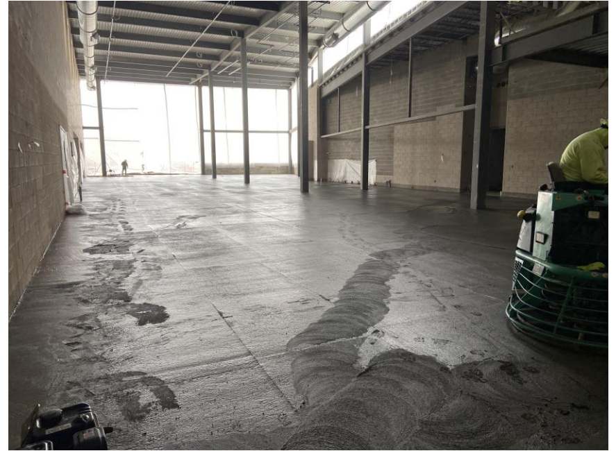
Concrete slab in commons area
