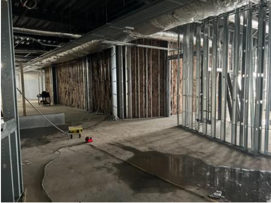
Drywall and insulation 2 nd and 3 rd floor
