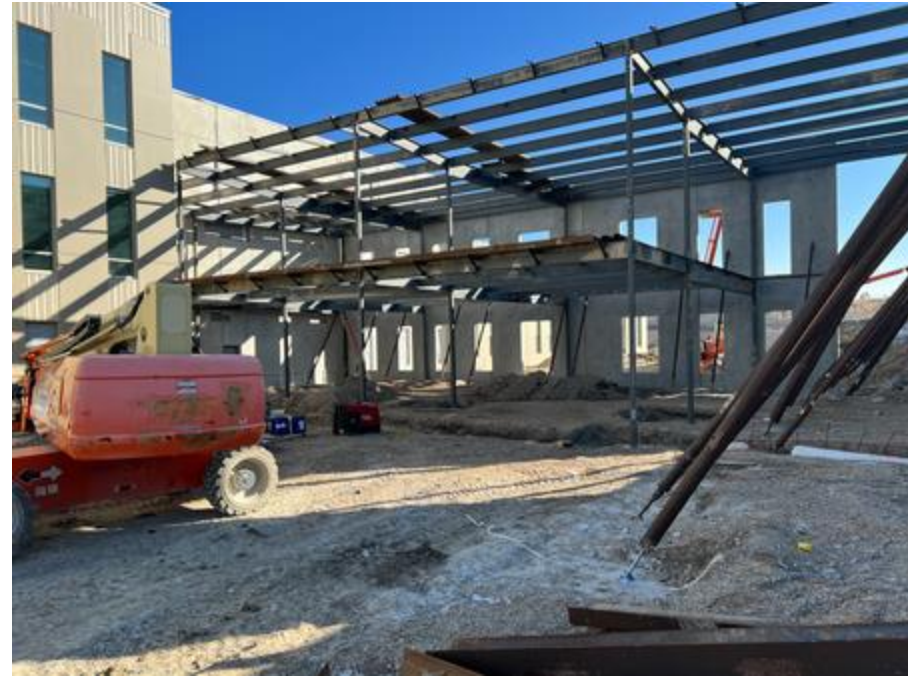
Steel stud and metal decking on the breezeway
