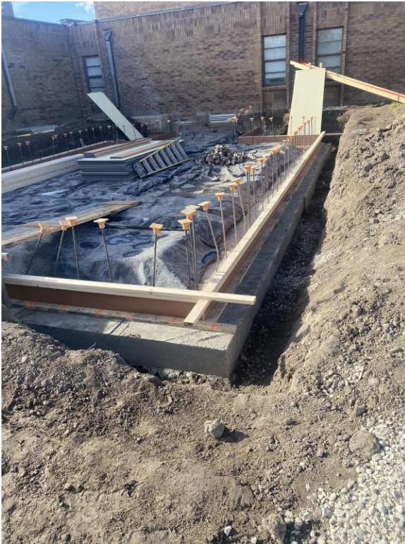
Mechanical room footings
