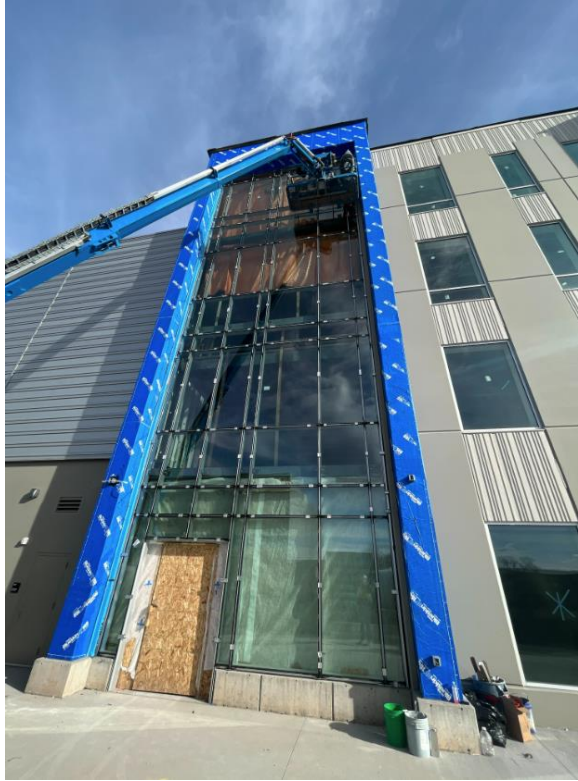
Glass being installed at the northwest stair tower of the main Academics Building
