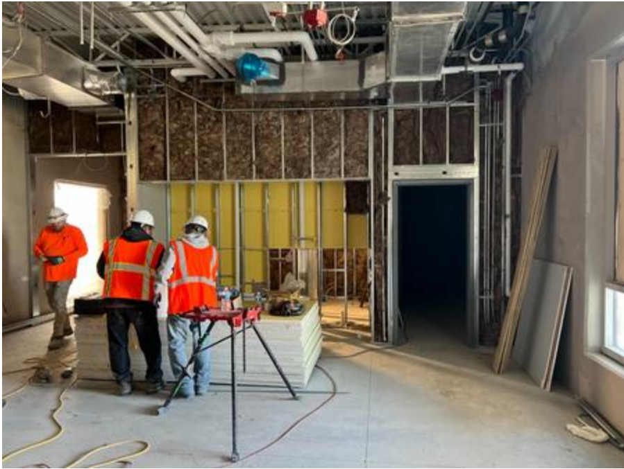
Locker room framing, drywall, and plumbing
