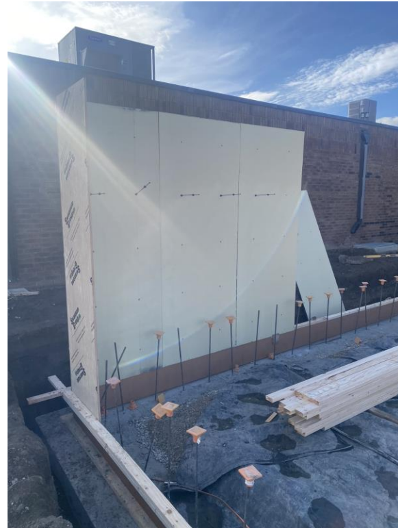
Concrete forms for walls
