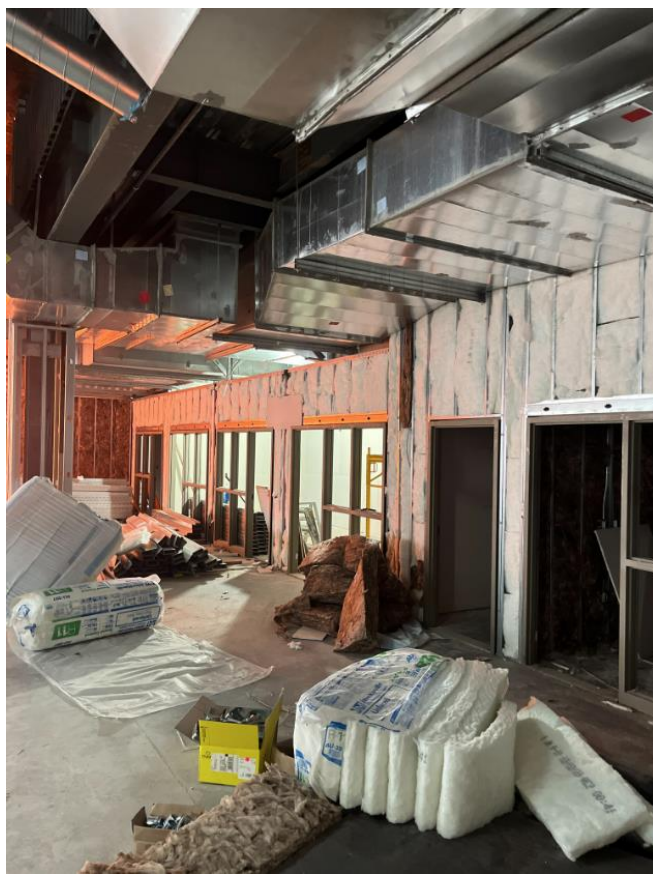
Media Center walls insulated, ready for sheetrock
