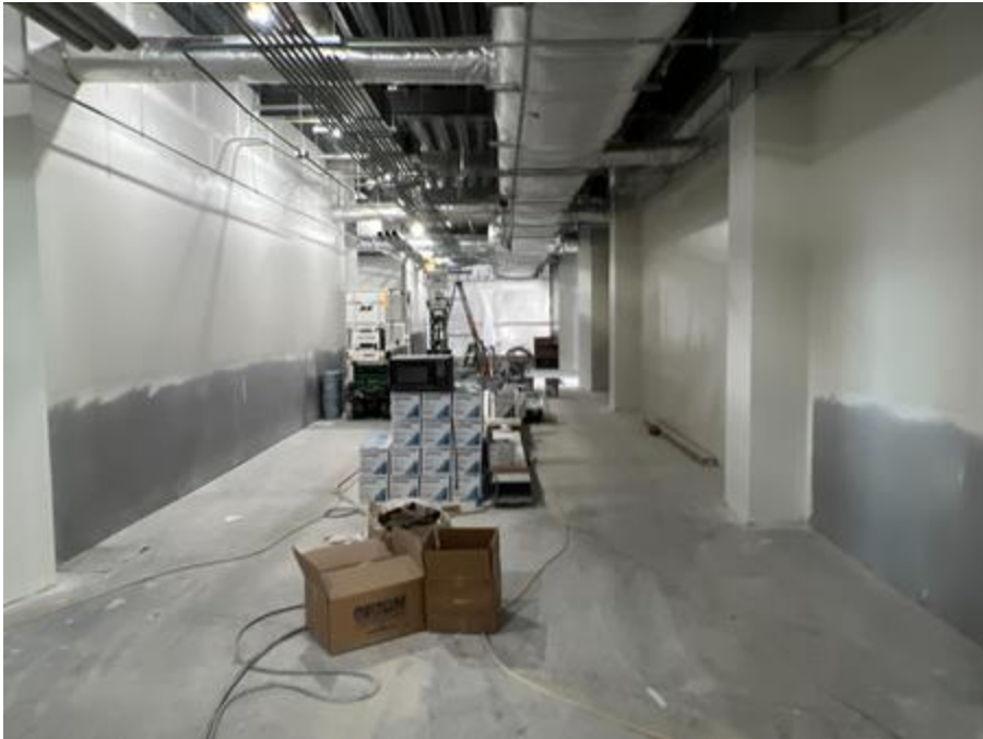
Paint and drywall 2 nd and 3 rd levels
