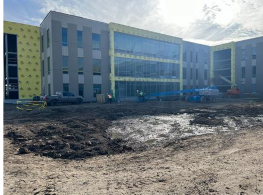
Curtain wall glass installation
