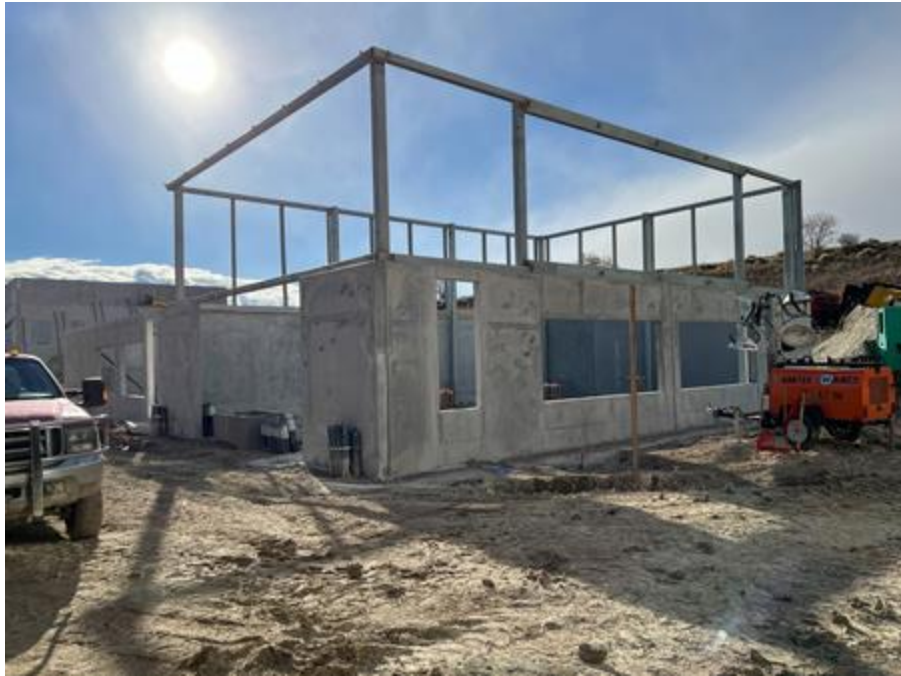
Mechanical yard tilt walls stood in place, steel erection
