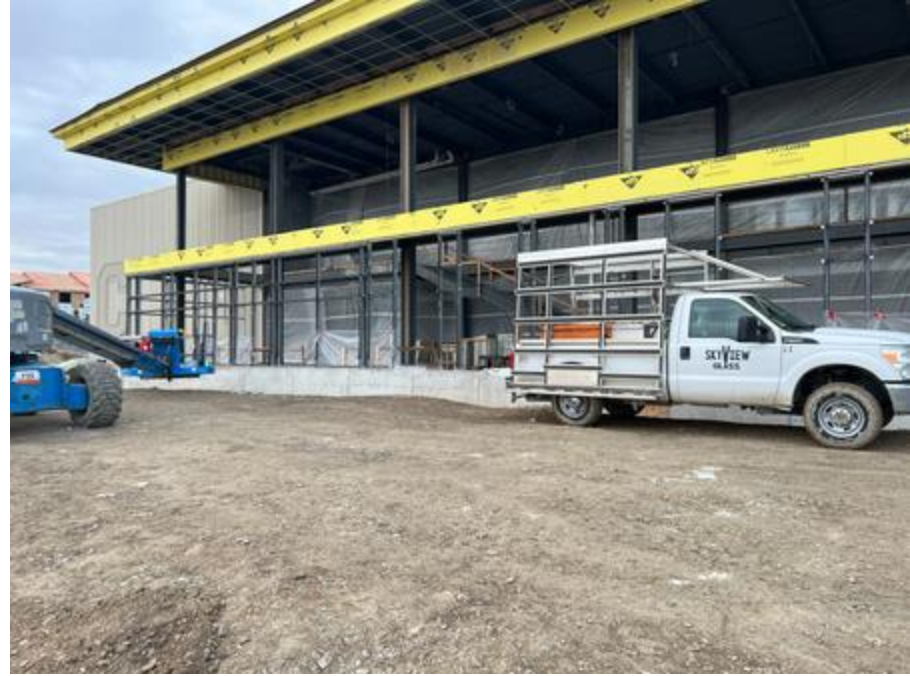
Vestibule curtain wall installation
