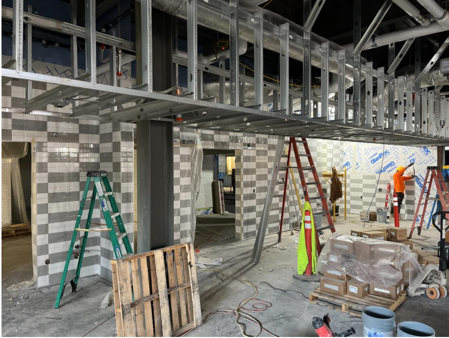
Tile being installed in the serving area of the Cafeteria
