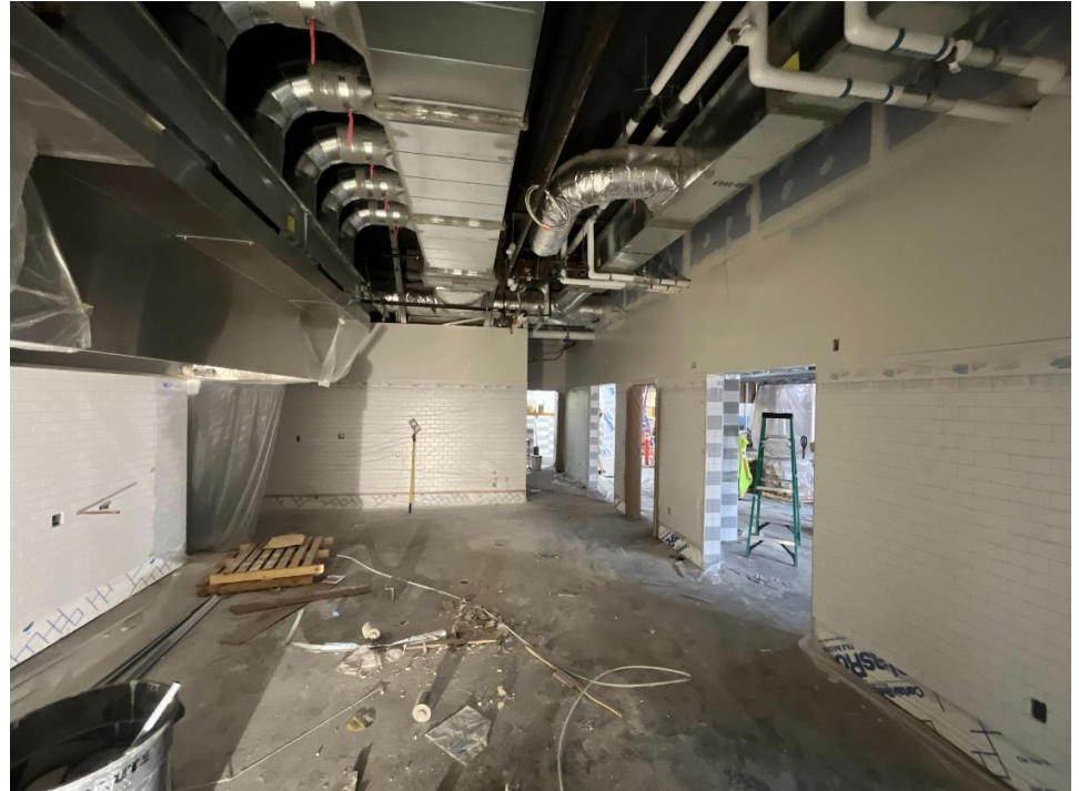
Kitchen being painted above the tile, getting ready for finish equipment
