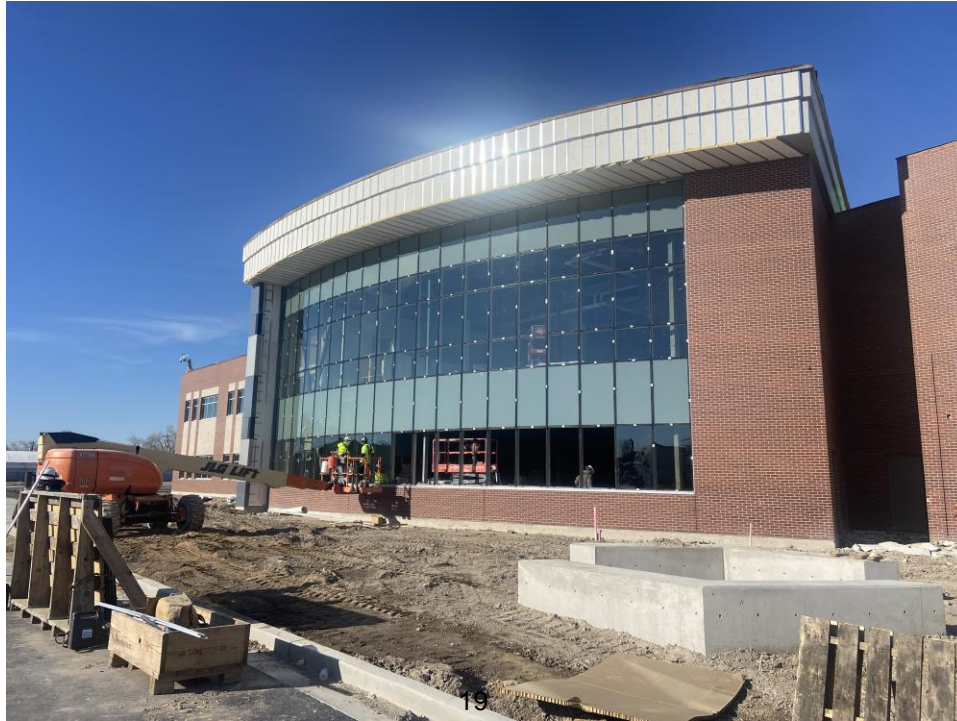
19 Glass installation at building exterior
