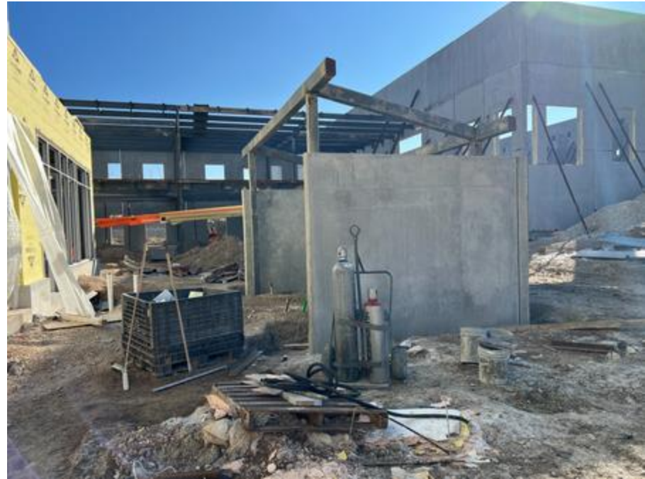
Exterior kiln walls stood into place
