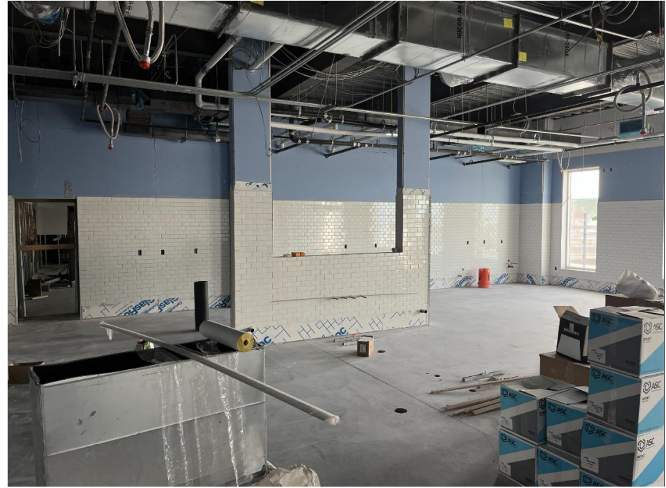
Tile installed in Culinary Arts classroom on Level 1
