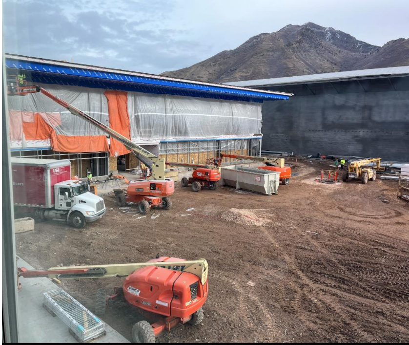
Curtain wall framing being installed on the south side of the Cafeteria
