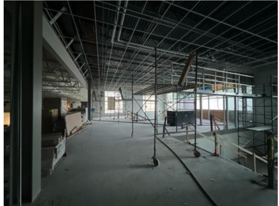
Drops ceiling grid level 1 of athletics
