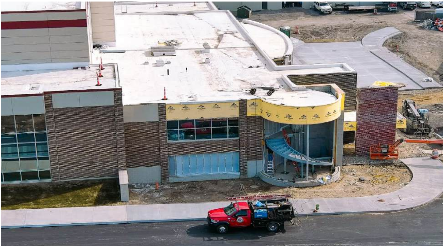
Construction Progress - November 2023
