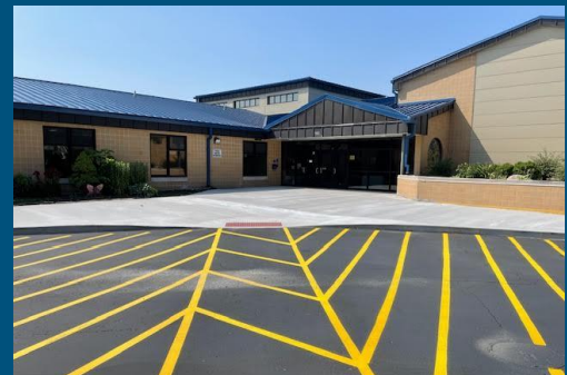
New Cement Work - Summer '24
