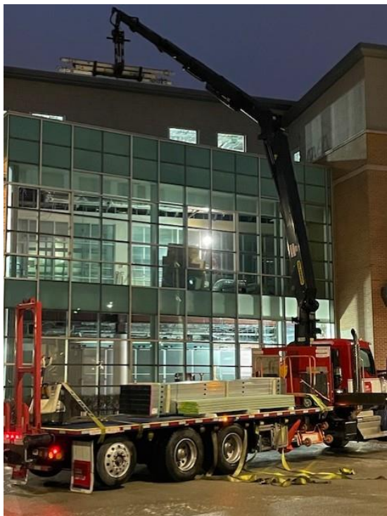
Left: Crane delivering sheet rock and dry wall for the 3 rd floor.
