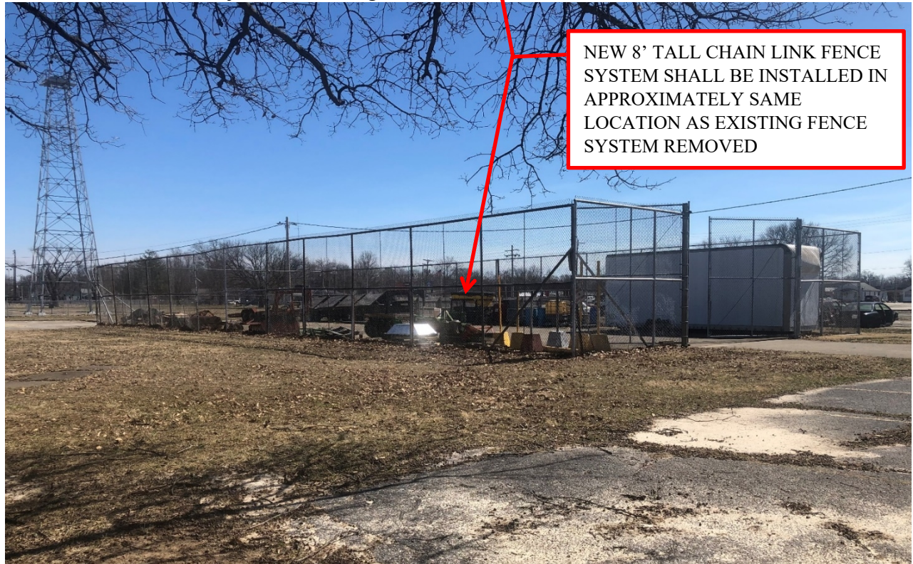
Northwest Corner of Project Site looking southeast
