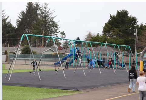
The new fall protection at Sam Case Elementary is complete.
