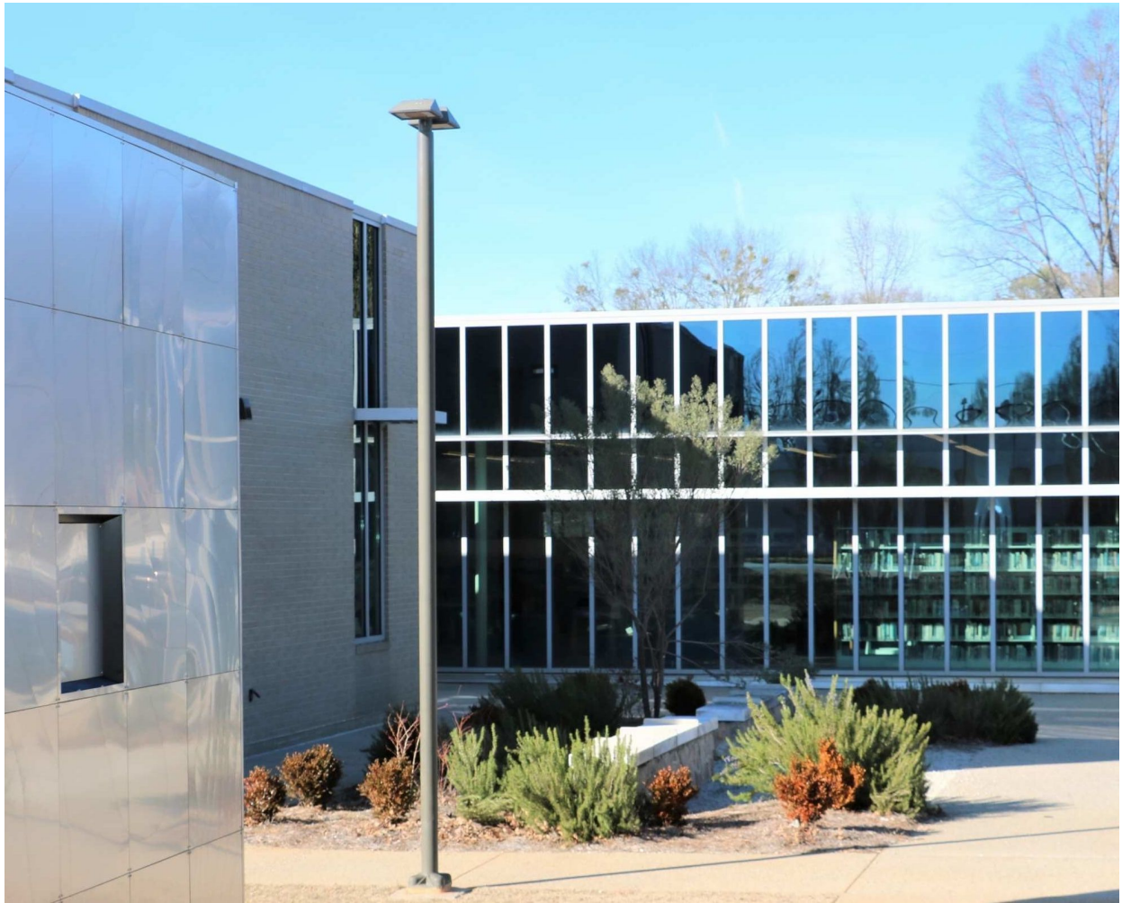
Metropolitan Library Resilience Hub, Fulton County GA
